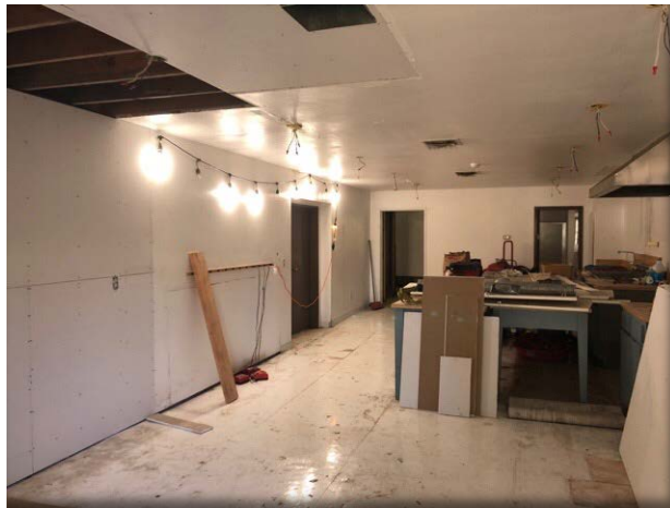
Office Associated with Hangar Mercer-Fraser
