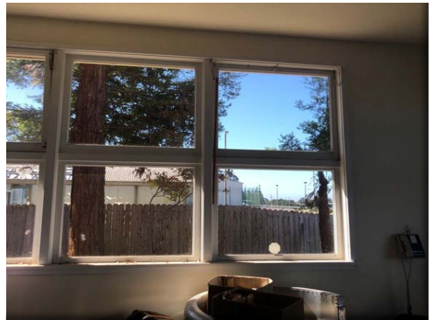
Office Associated with Hangar Mercer-Fraser
