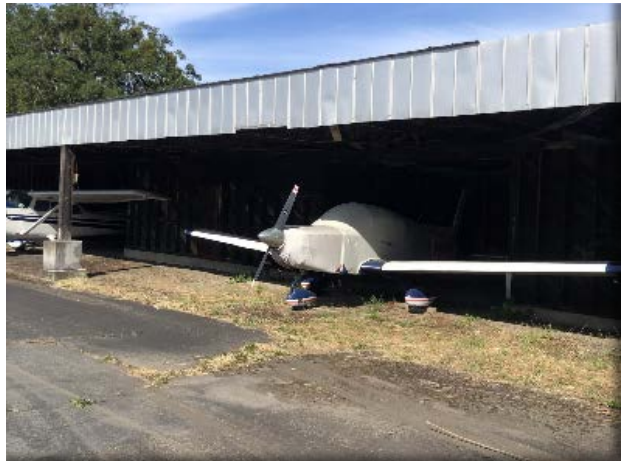
Small T-Hangar (O16)
