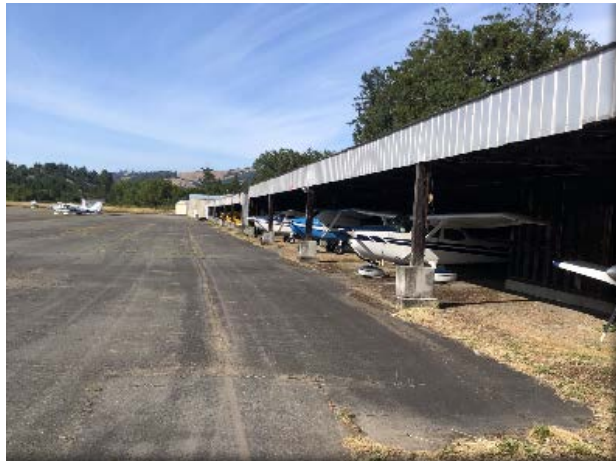
Small T-Hangar (O16)
