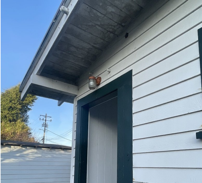
Figure 8: Non-Conforming Outdoor Lighting To be Replaced
