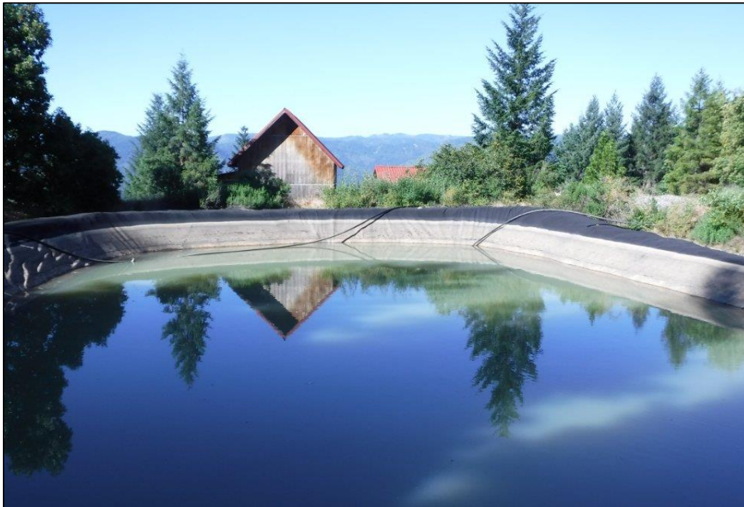
Photo 3. Off-channel, rainwater catchment pond that provides irrigation water for APN 524-112-002 during the forbearance season. This will be retrofitted with semi-floating dock for to allow any animals to exit the lined-pond.
