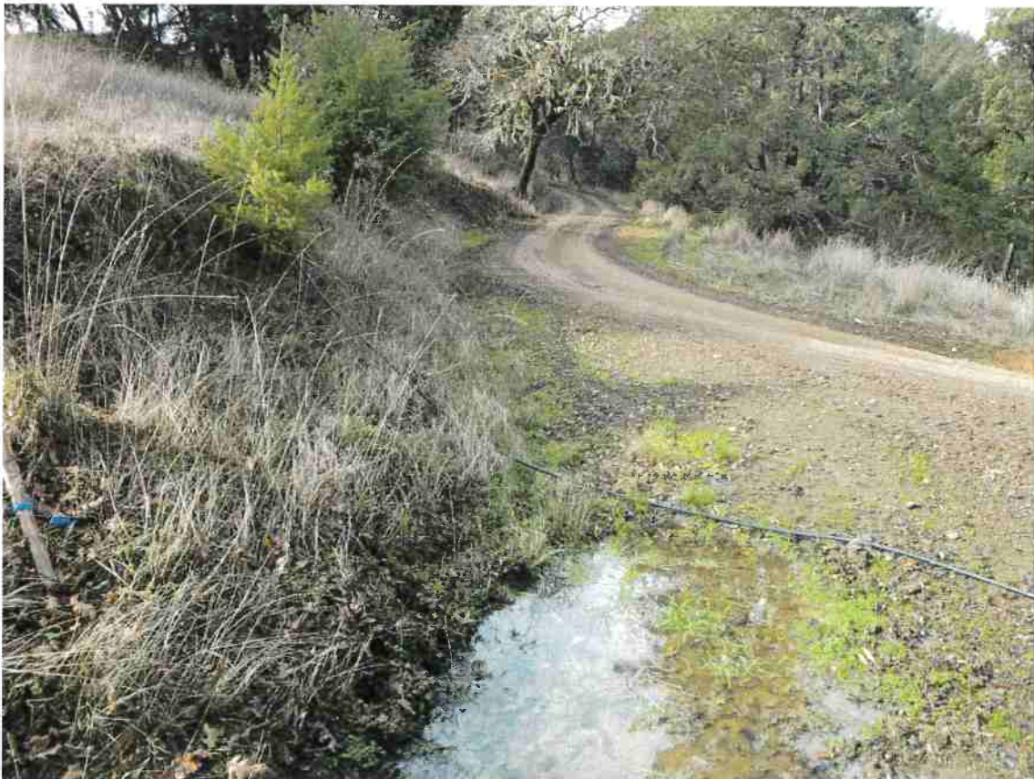
Photo 14. Looking upslope at Road 1 inboard ditch from intersection with Road 2
