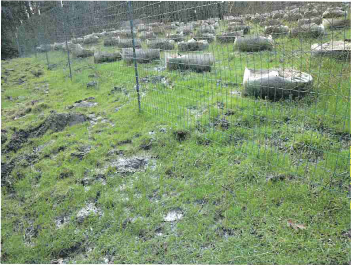
Photo 11. Lower slope of North Cultivation with water percolating through surface. 1/10/19
