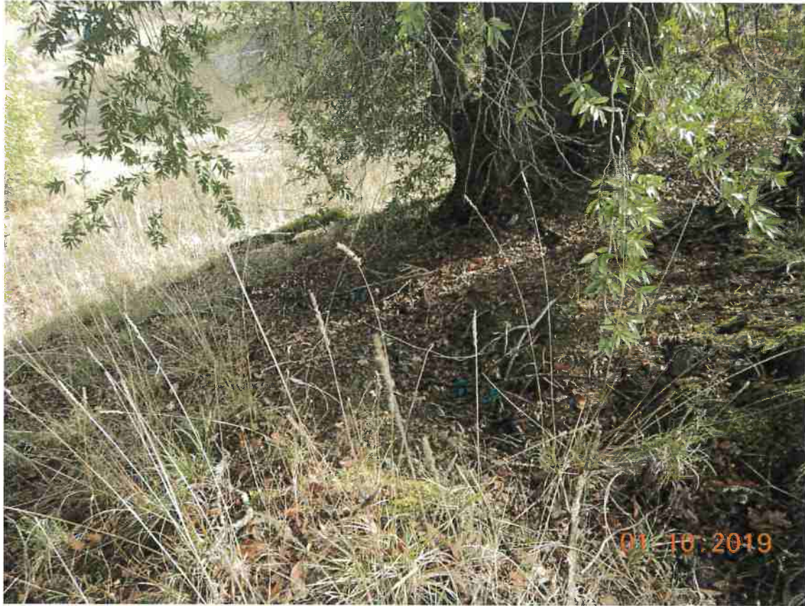
Photo 15. Looking down ditch where pooled water from Photo 14 should drain
