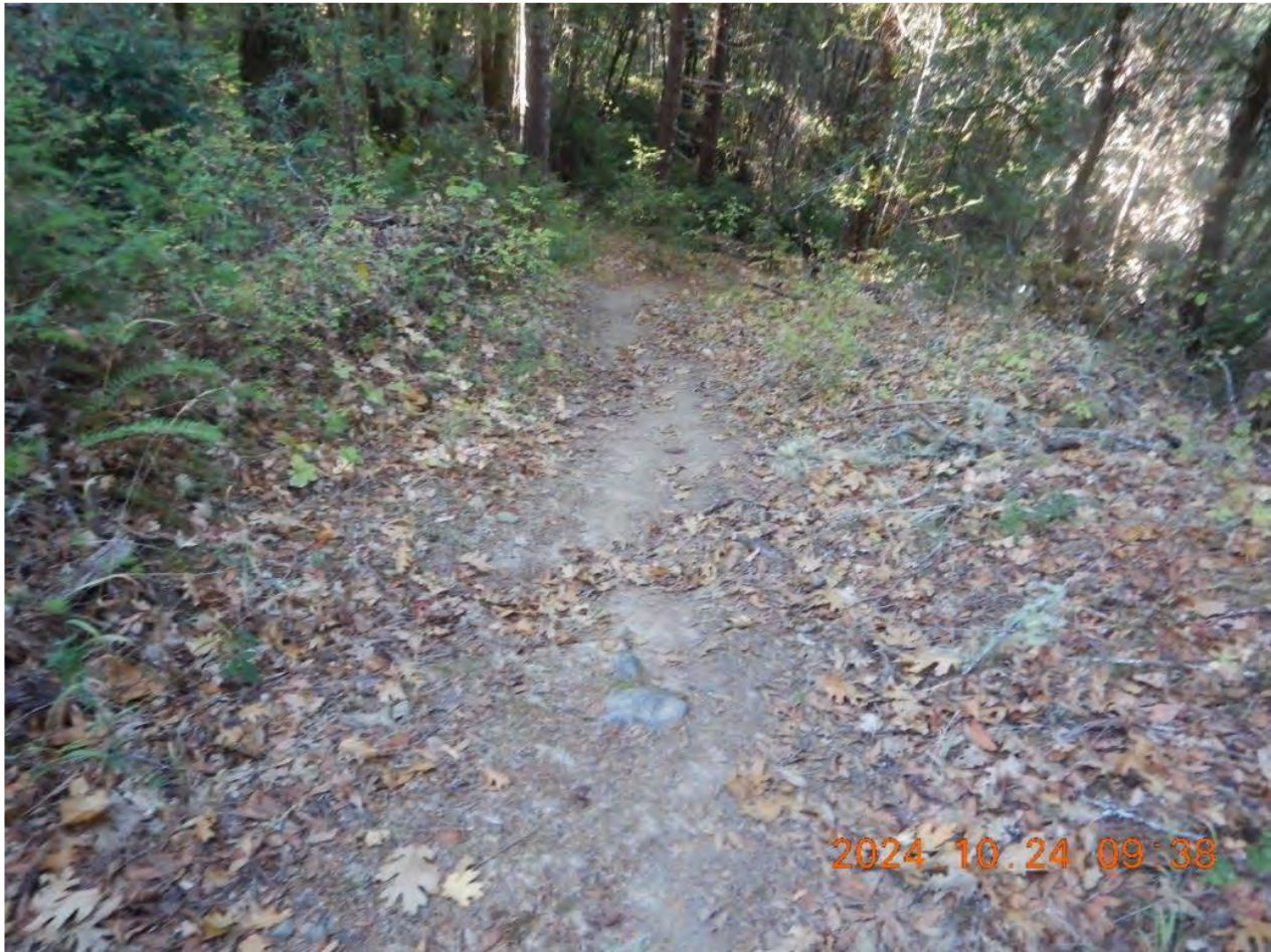
Fig. 3.1 Water bar needs to be reinforced. Photo by NCRWQCB, 24 October 2024.
