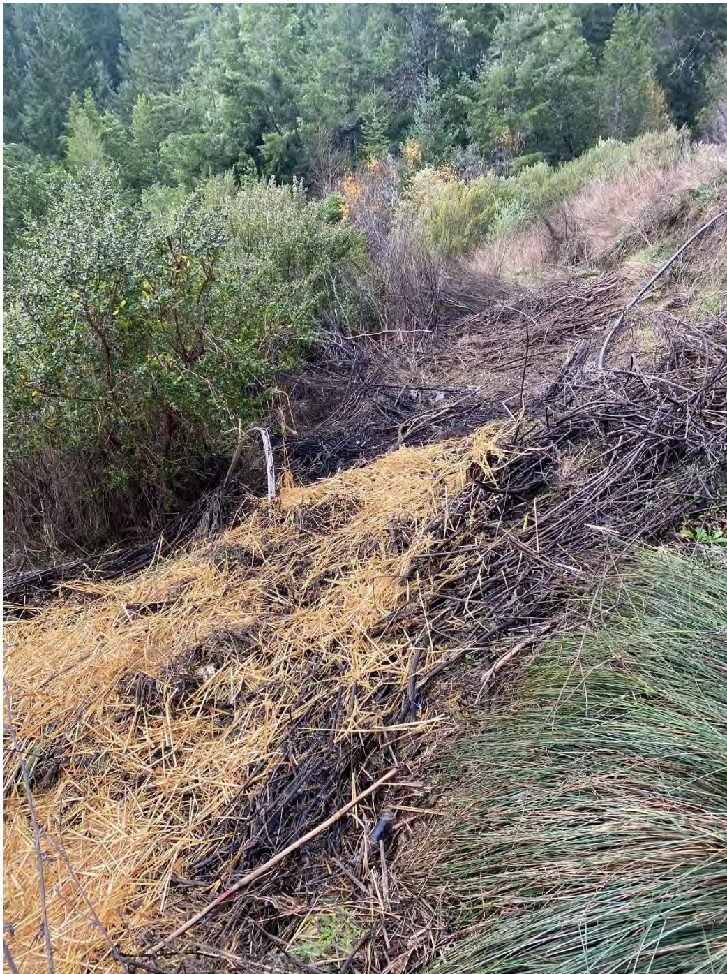
Fig. 6.3 Erosion control implemented at fill slope near CA2. Photo by Permittee, 20 December 2024.
