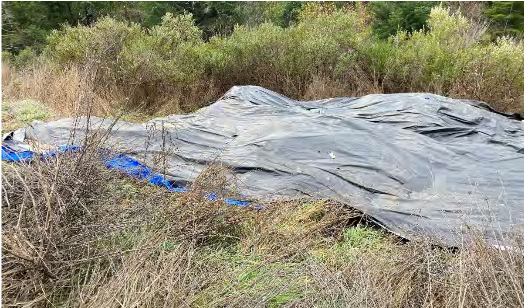
Fig. 5.3 Potting soil covered on fill slope of the graded flat at CA2. Photo by Permittee, 20 December 2024.
