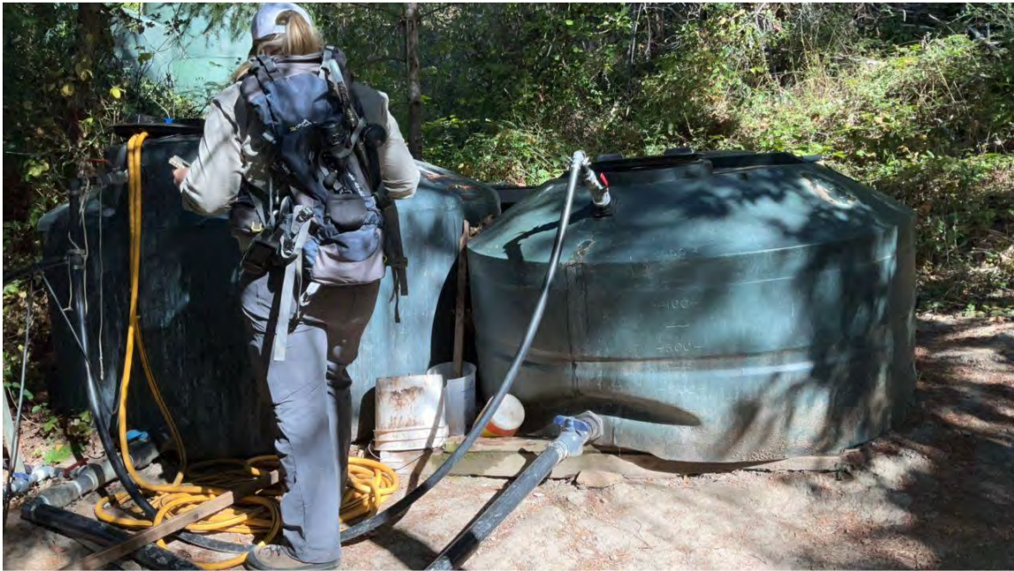
Fig. 16.1 The surface water diversion line from Point 2 connects to water storage tanks above CAI at Point 16 and appears to be used to irrigate. Photo by NCRWQCB, 24 October 2024.
