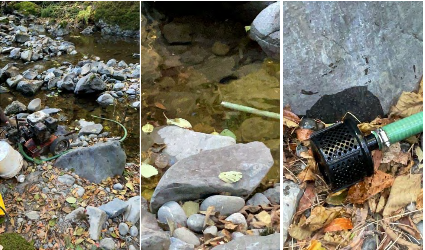
Figs. 2.3-5 Surface water point of diversion, intake, and screen in Little Larabee Creek. Photos by NCRWQCB, 24 October 2024.
