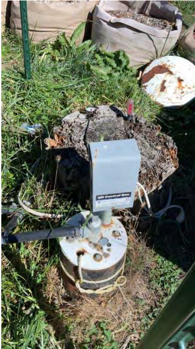
Fig. 13.1 Well located at Point 13, within the cultivation area CA1. The well was unplugged. Photo by NCRWQCB, 24 October 2024.
