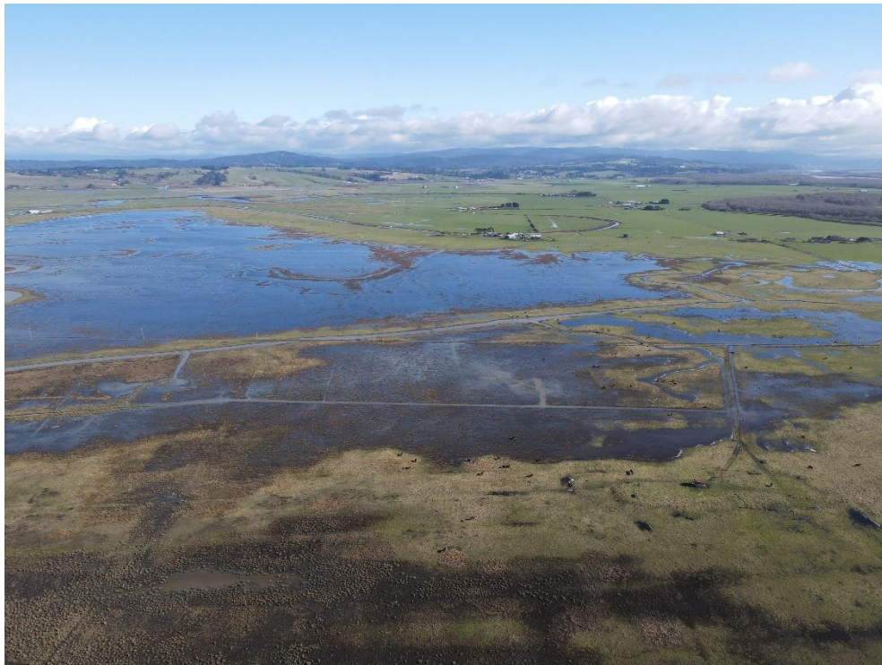
Photo 2—Drone footage from December 2021, looking east at muted tidal flooding that occurs within the interior of the existing levees, namely within the NRCS Wetland Reserve Easements (WRE). The small sliver of dry land in the furthest eastern extent of the Project Area is on private property that is proposed to be protected behind the new levee construction.
