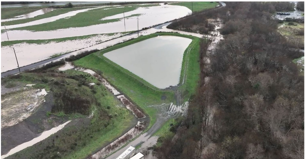
The unpermitted stormwater impoundment facility
