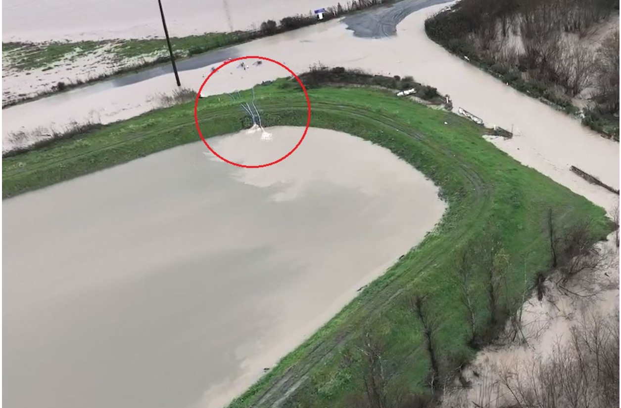
Pumps running to collect stormwater from the lower yard into the impoundment feature.
