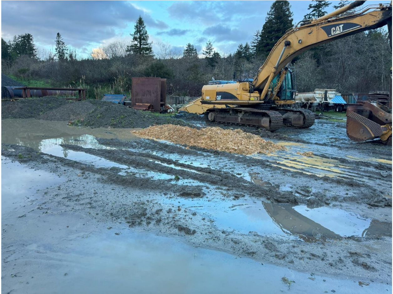
Picture 10 – View of fine clay sediment material (light colored material in picture) that was stockpiled on the ground in the lower yard. This entire area was exposed to rain and no sediment and/or erosion control BMPs were observed. Picture taken by Walt Dragaloski.
