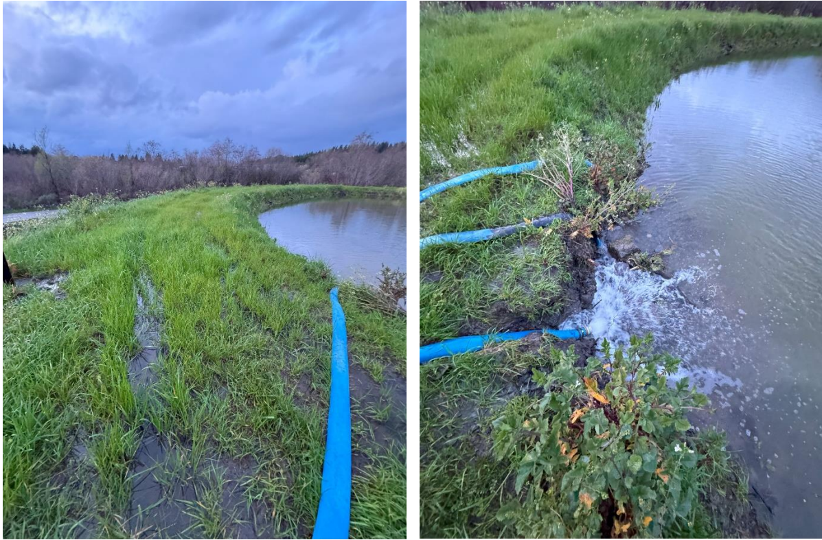
Picture 14a and 14b – The left picture shows the hose used to pump the stormwater from this retention pond in the lower yard to the infiltration trenches in the upper yard. The right picture shows the three hoses used to pump stormwater from the swale shown in the previous picture into the retention pond. Picture taken by Walt Dragaloski.
