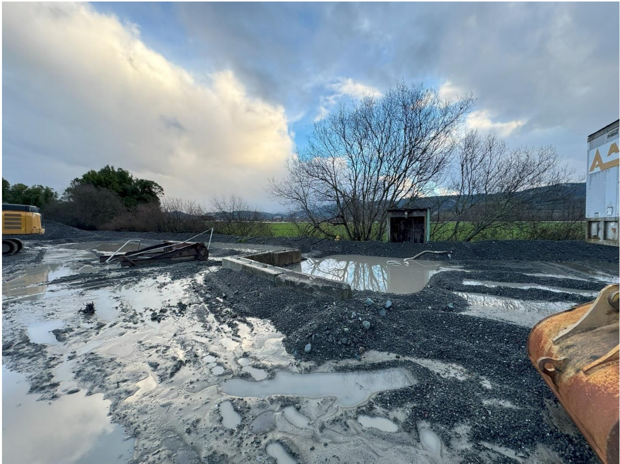
Picture 4 - View of sediment trap at the southern portion of the upper yard. The adjacent upper yard area flows through this sediment trap to the infiltration trench inlet. A thick layer of sediment was observed on the ground within the sediment trap. Additionally, a sheen was observed on the water surface and a black residue stain was visible in this area. This sediment trap drains the turbid water into the infiltration trench. Minimum BMPs were not observed within this area. Picture taken by Walt Dragaloski.
