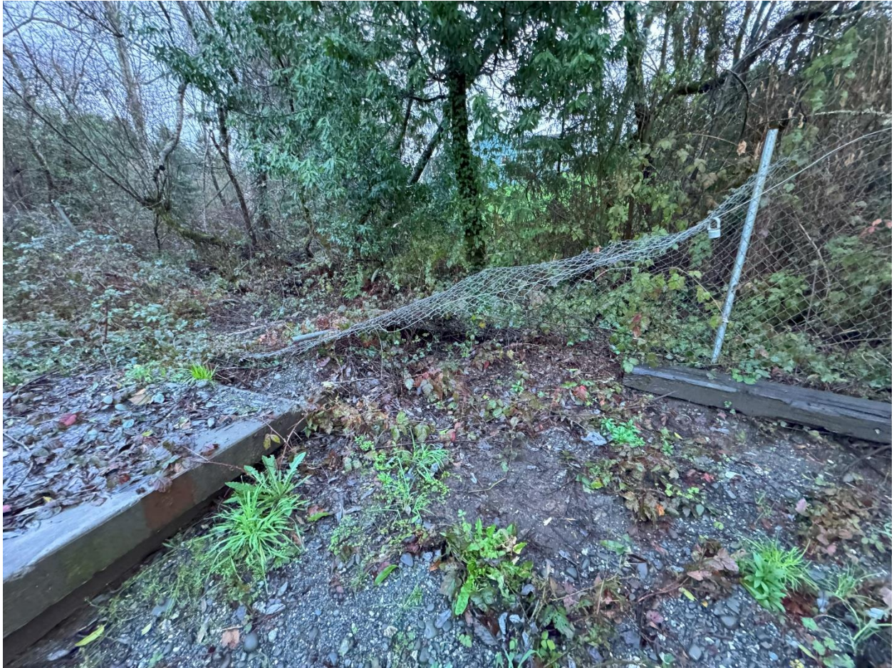
Picture 11 - View of damaged fences adjacent to Noisy Creek along the eastern boundary of the Facility in the lower yard. Evidence of erosion due to concentrated flow towards Noisy Creek was observed near the fence line, corroborating observation of stormwater discharge from the Facility to Waters of the State by the adjacent homeowner. Picture taken by Walt Dragaloski.
