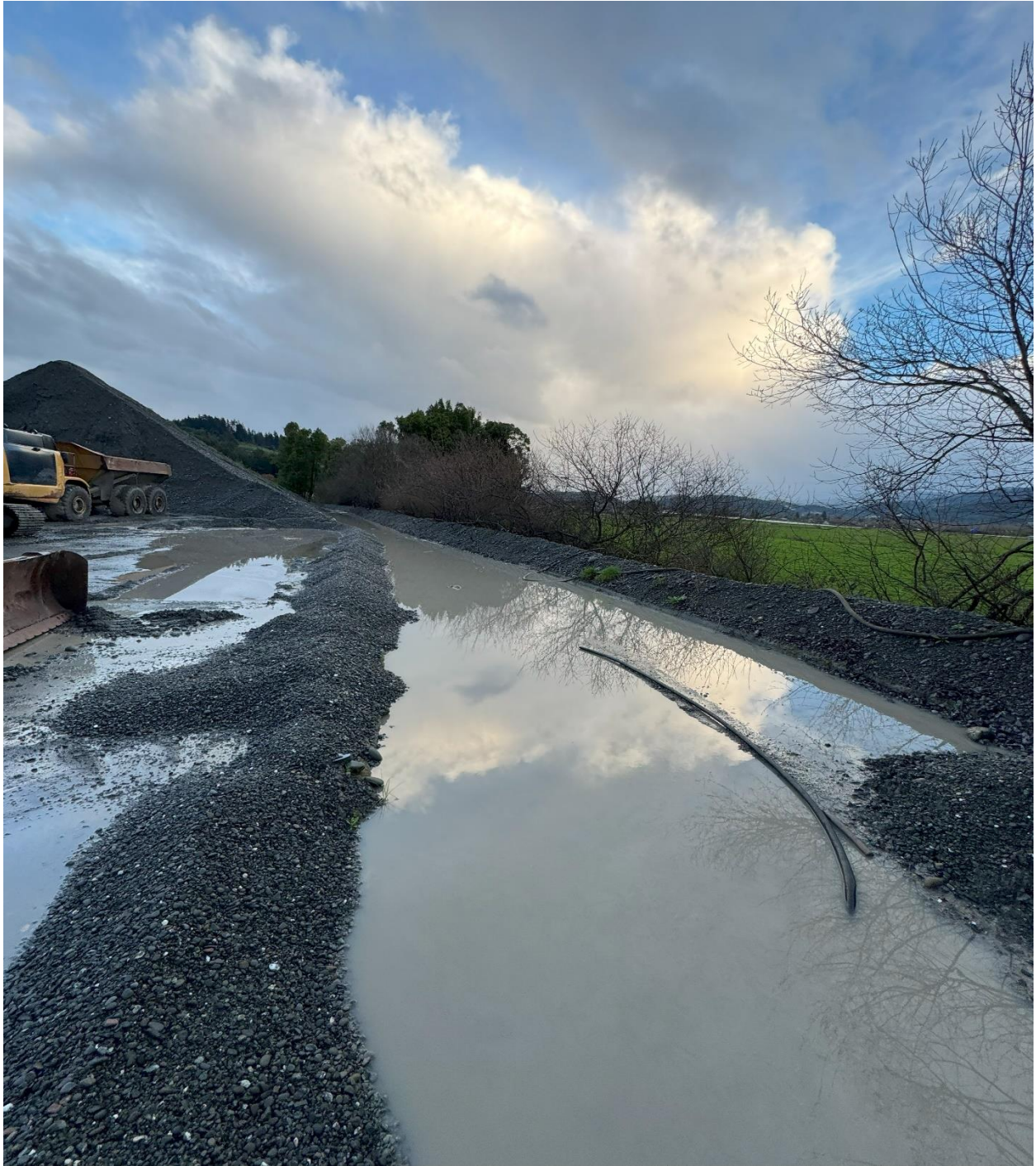
Picture 3 – Looking east at accumulated turbid stormwater along southern portion of the upper yard flowing to infiltration trench inlet. Picture taken by Walt Dragaloski.
