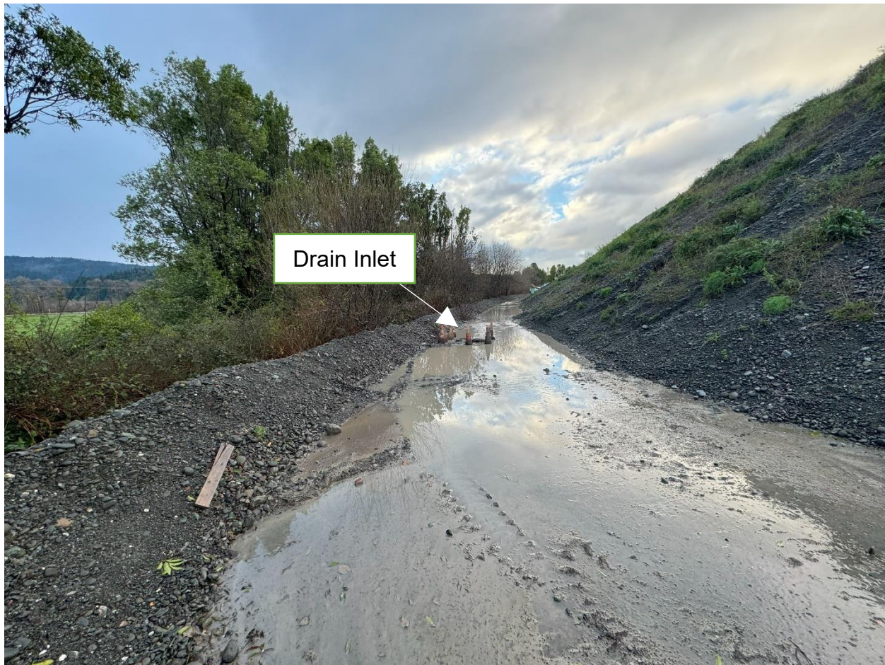
Picture 2- View of a large and uncovered aggregate stockpile located in the Upper Yard. Accumulated turbid runoff was observed around the stockpile within this muddy area. The runoff from this area drains to the infiltration trench via an infiltration trench inlet. Picture taken by Walt Dragaloski.
