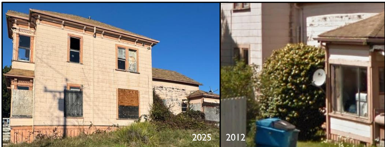
Figure 9: Church Street Façade, Prior Conditions, 2025 and 2012.
