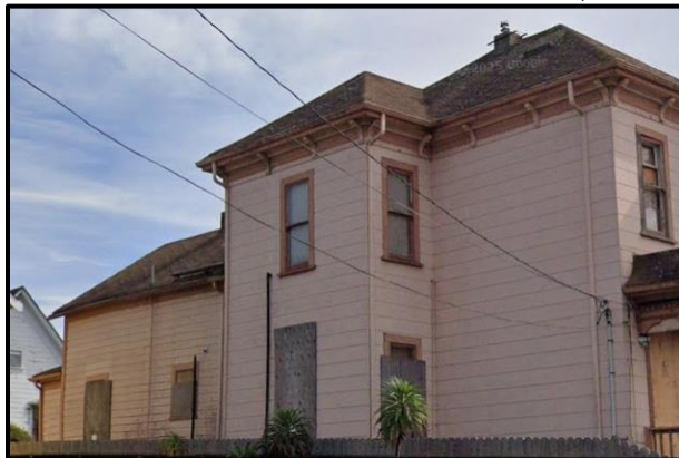
Figure 15: Interior Lot Line Façade, Prior Conditions, 2024.
