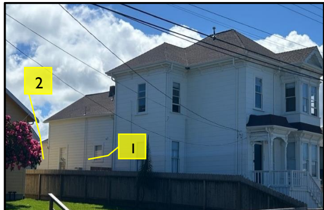
Figure 16: Interior Lot Line Façade, Post-Rehabilitation, 2025. View from Street (upper) and View from Alley (lower).
