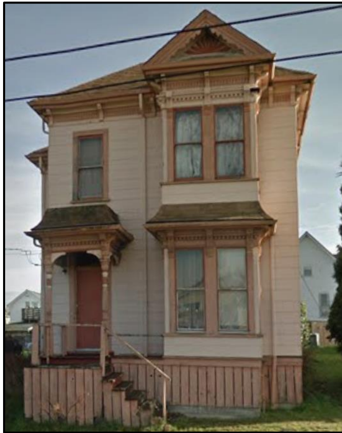
Figure 4: Pine Street Façade, West Elevation, 2011.
