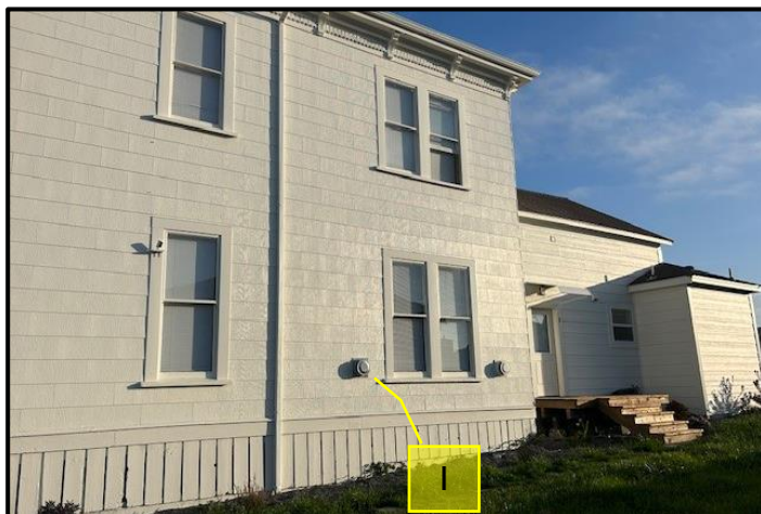
Figure 10: Church Street Façade, Post-Rehabilitation, 2025.
