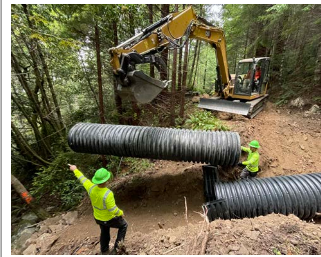
Upgraded replacement of a 30" culvert with new 36" culvert in JCF (as part of NTO #24; Crossing X-B)
