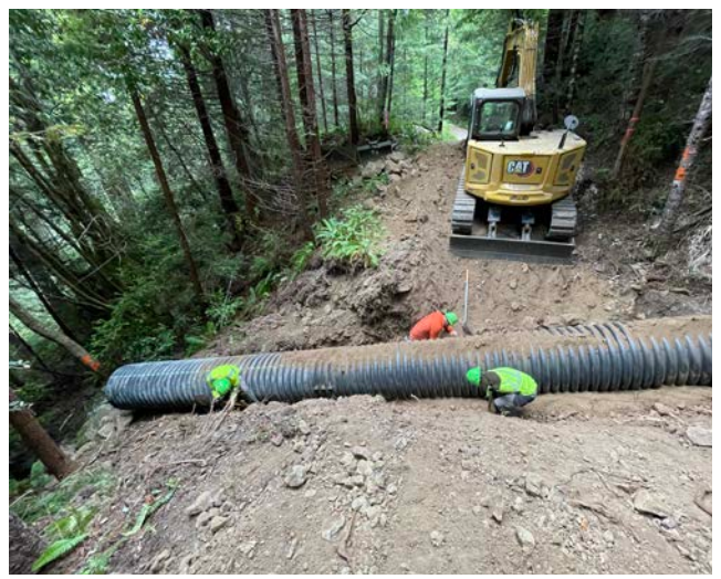
Upgraded replacement of a 30" culvert with new 36" culvert in JCF (as part of NTO #24; Crossing X-B)
