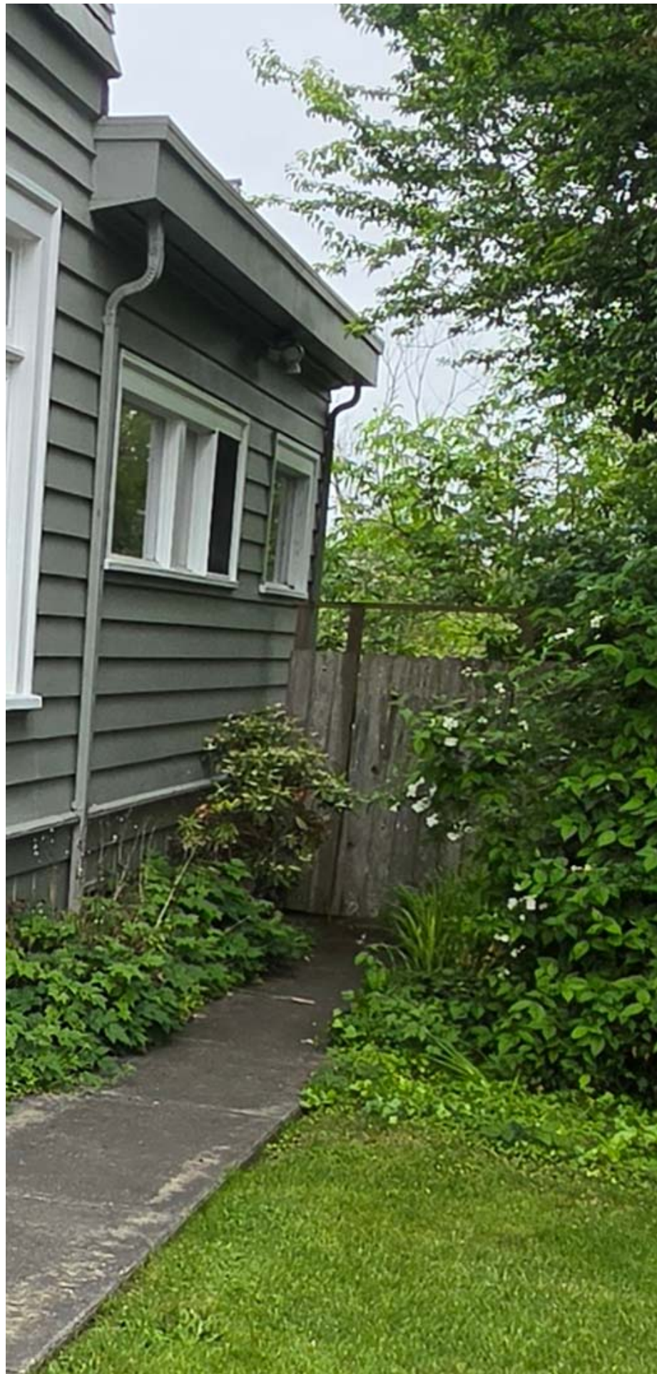
3 EXISTING KITCHEN EXTERIOR NO SCALE
