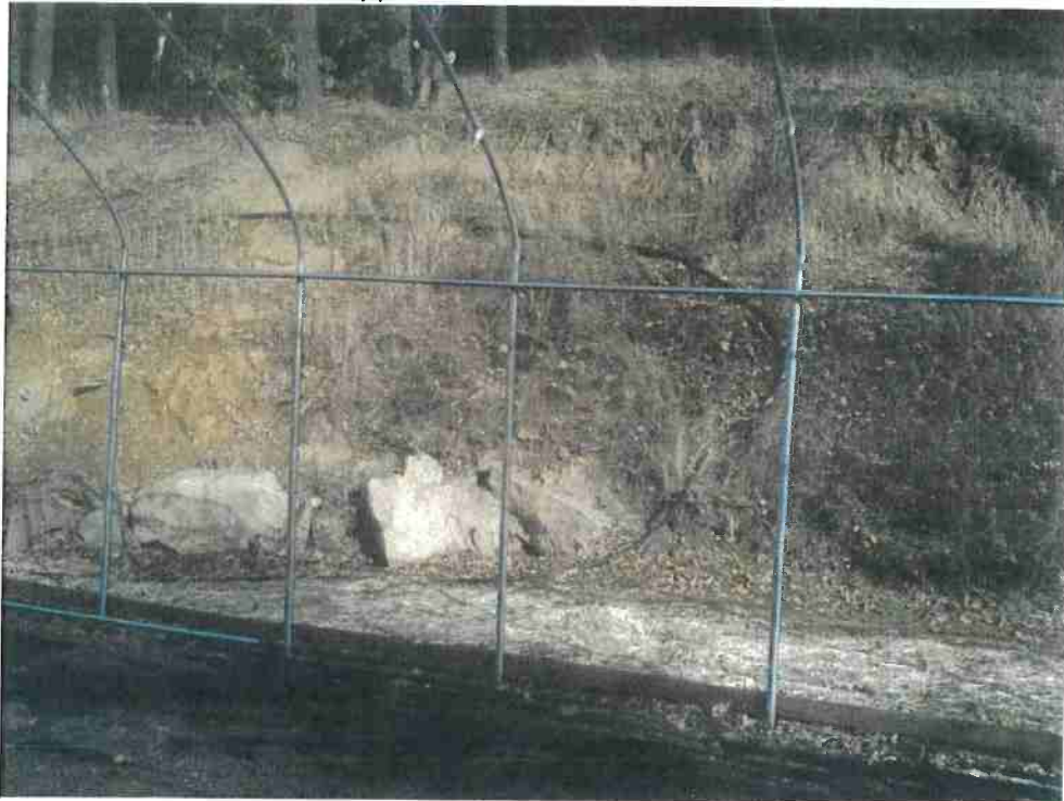
Figure 2 Upper terrace Cut Bank Failure
