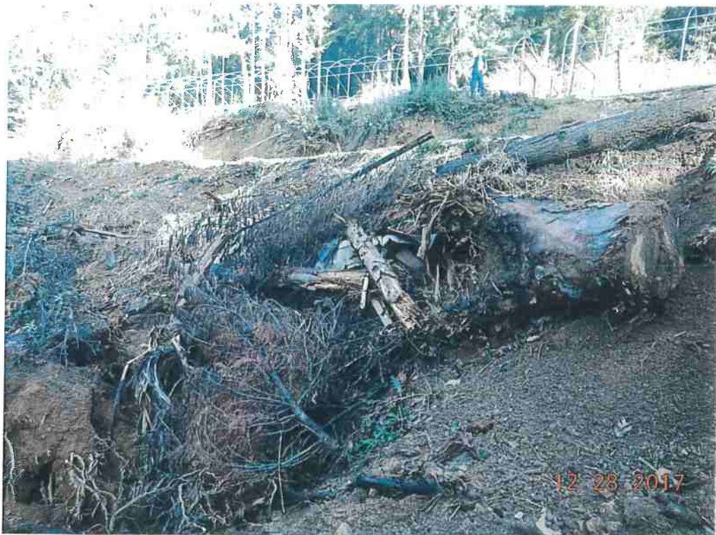
Figure 6 Lower Terrace Fill Slope
