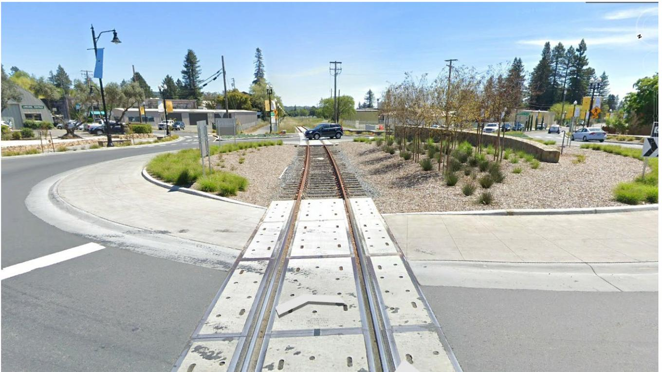
Image 1 – Example of a roundabout that accommodates railroad use in Healdsburg, CA at Mill and Vine Streets (image via Google Earth Street View)
