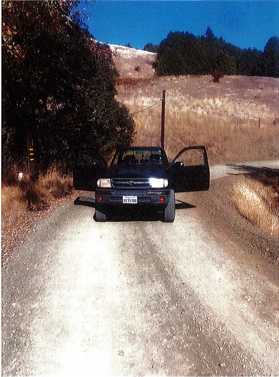
Figure 15: RP-15. Road width: 15' 3".
