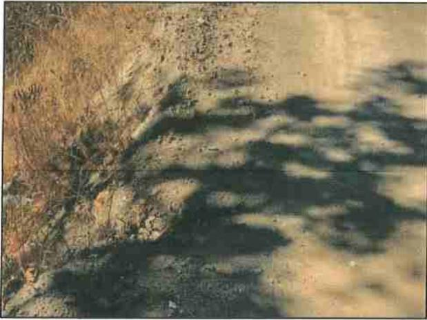
Photo #145 River Rd Looking @ Erosion Issue From Lack of Functioning Culvert
