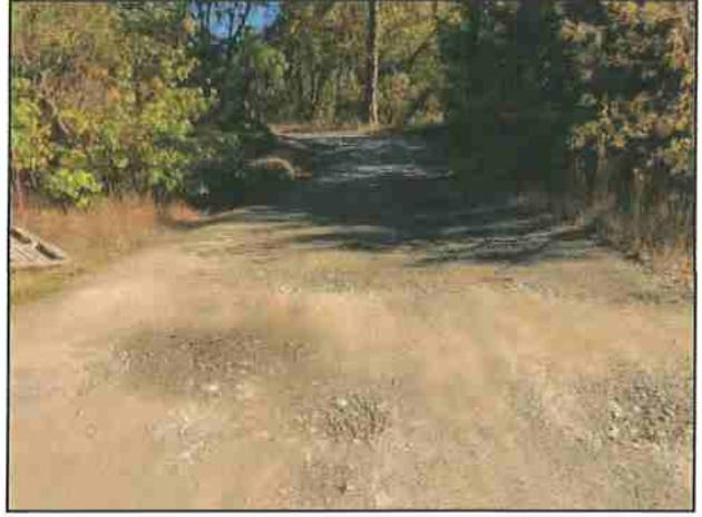
Photo #14 River Rd Looking SE @ Potholing Caused by Poor Drainage
