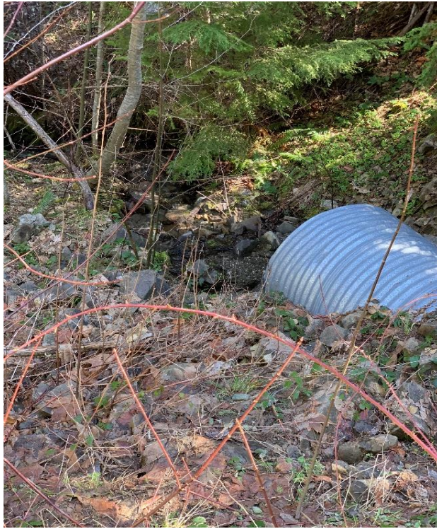
Figure 3: RP 3 on Supply Creek Rd. - Culvert (side A)
