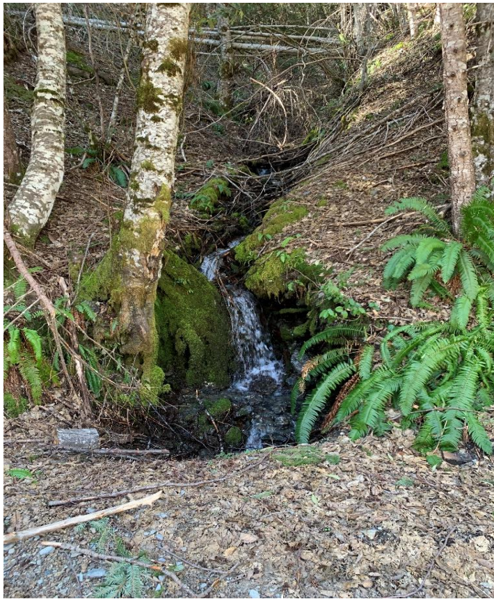
Figure 7: RP 5 on Supply Creek Rd. - Culvert (side A)
