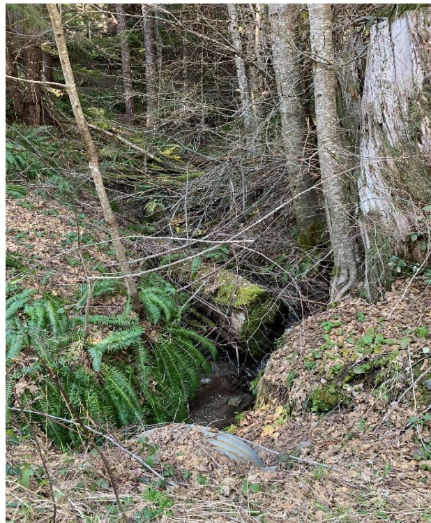
Figure 4: RP 3 on Supply Creek Rd. - Culvert (side B)
