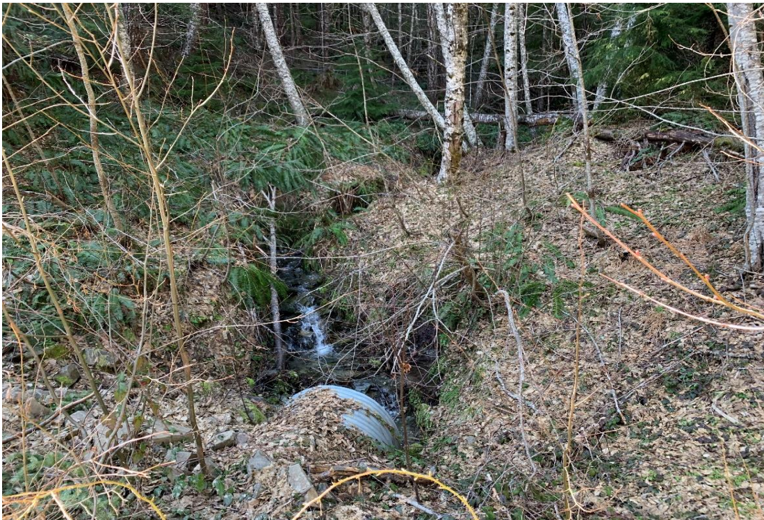
Figure 8: RP 5 on Supply Creek Rd. - Culvert (side B)
