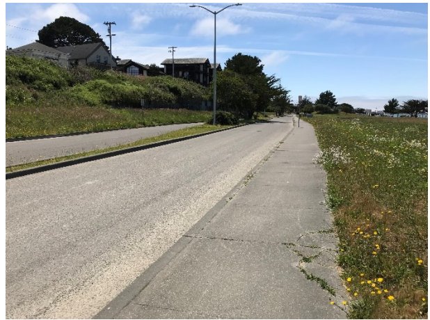
Existing Conditions Waterfront Drive: No room for bike lanes.
