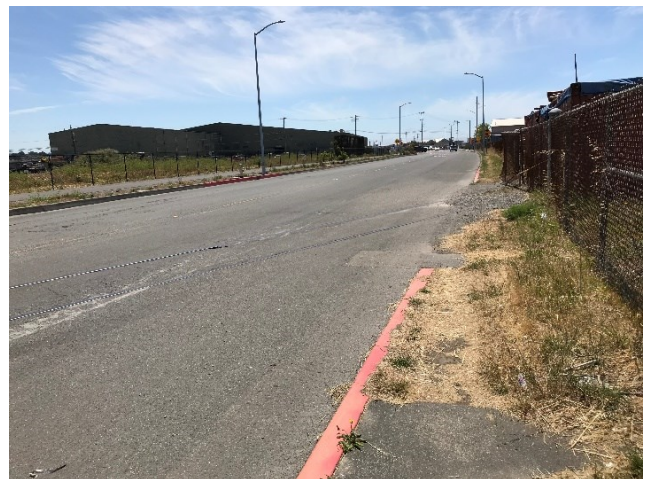
Existing Conditions Waterfront Drive: No sidewalk facilities/sidewalk gaps
