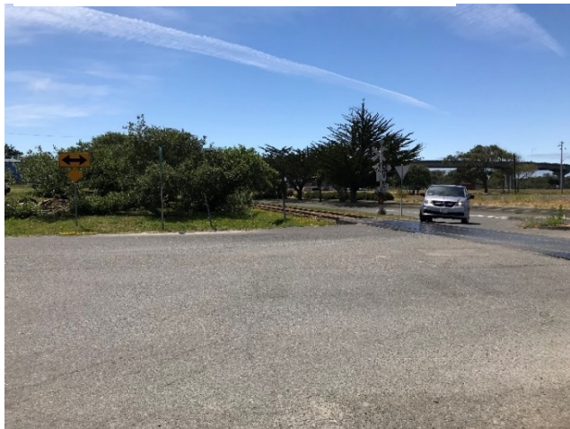
Existing Conditions: Realignment Section: Poor intersection lay out
