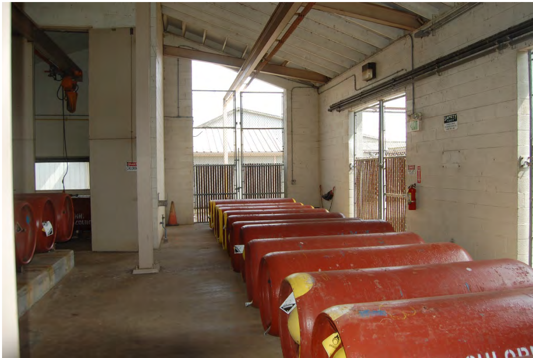
Photo 51 - Chlorine Storage Building
