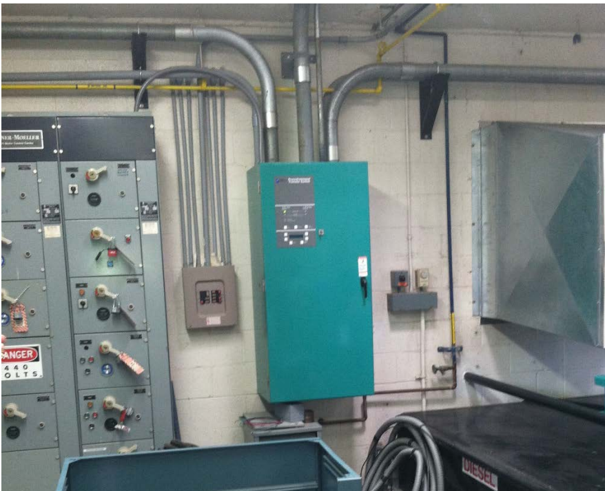
Photo 63 - Transfer Switch
