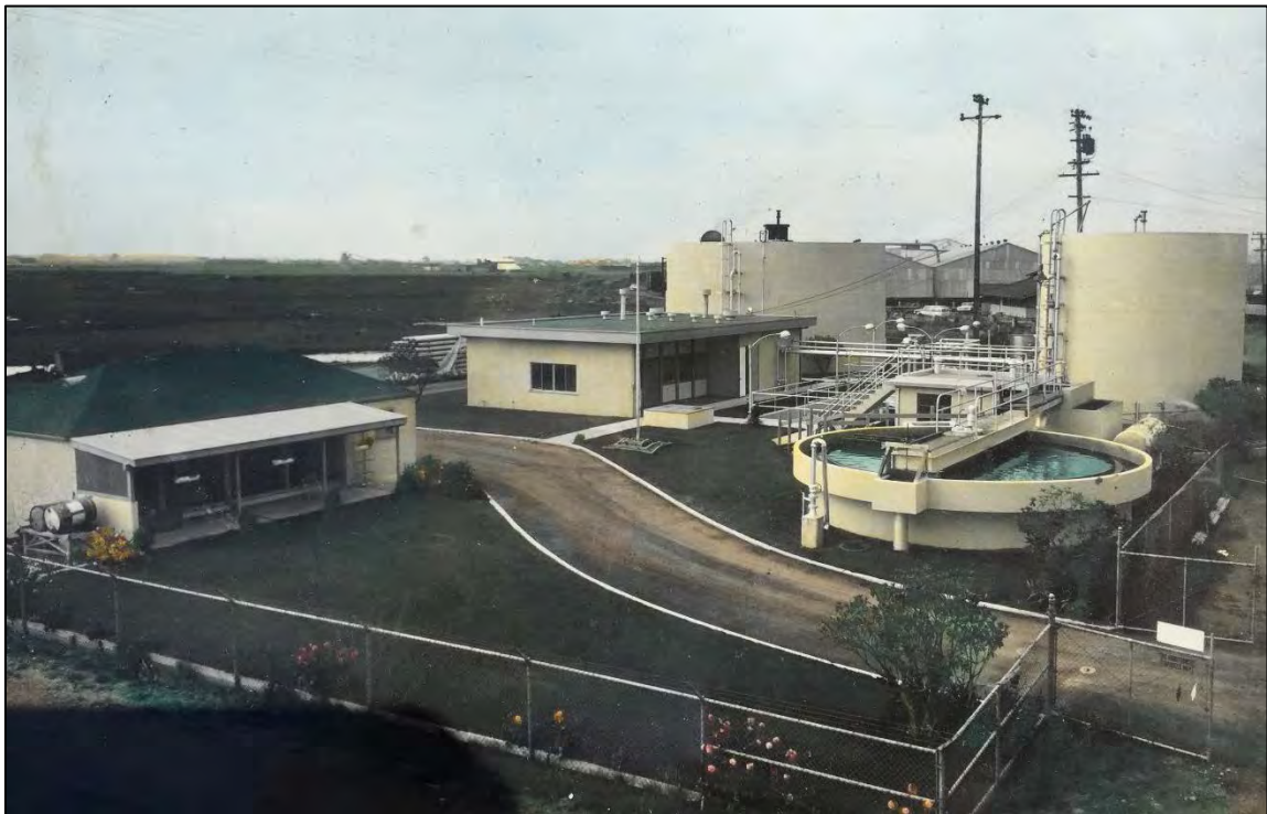
Figure 5.1 Original Arcata Wastewater Treatment Plant (Circa 1958)
