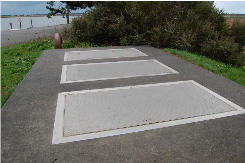
Photo 44 - Hauser Effluent PS - Pump Station Vault
