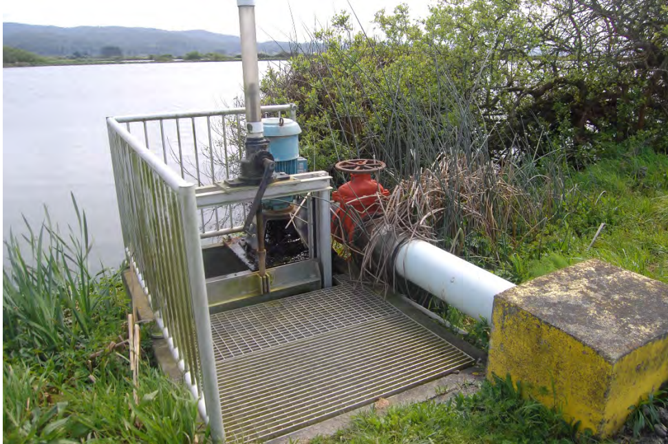
Photo 31 - Treatment Wetlands Influent Box - Wetlands 4 feed pump
