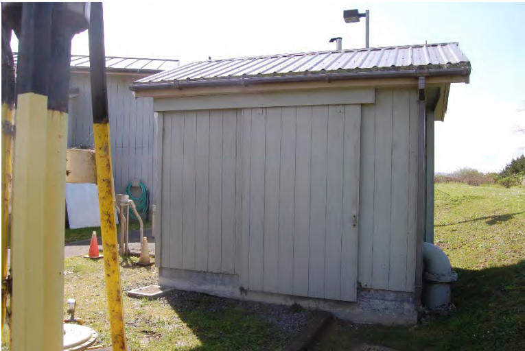
Photo 38 - Emergency Pond Pump Station
