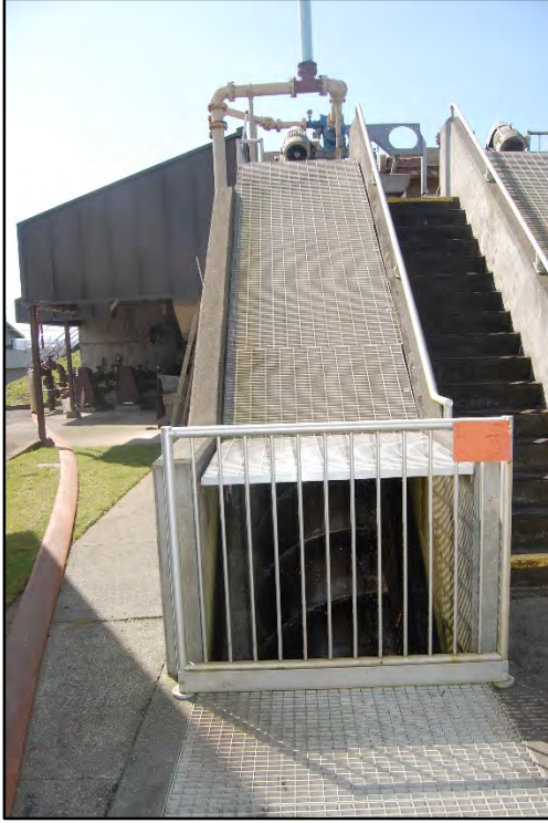
Photo 03 - Headworks - Facing the Archimedes Screw Pumps
