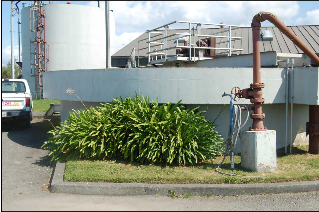
Photo 15 - Primary Clarifier No. 1
