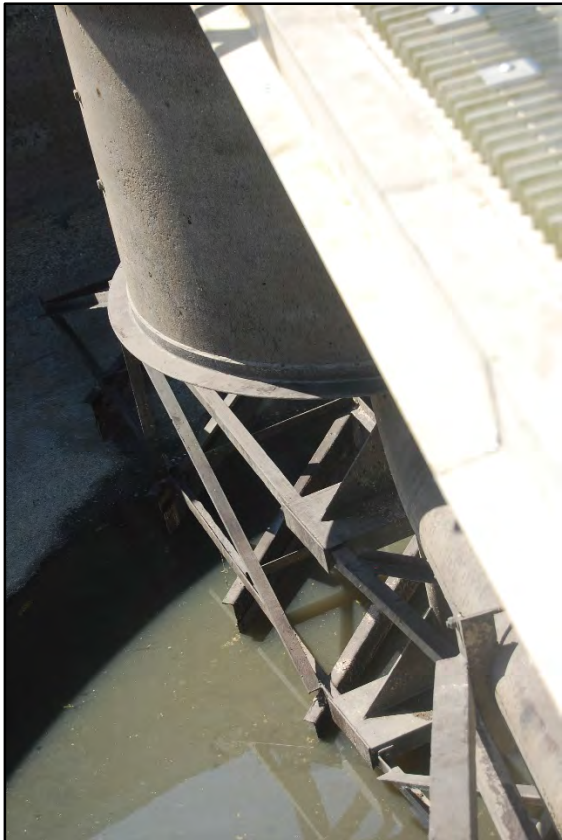
Photo 18 - Primary Clarifier No. 1 - Mechanism
