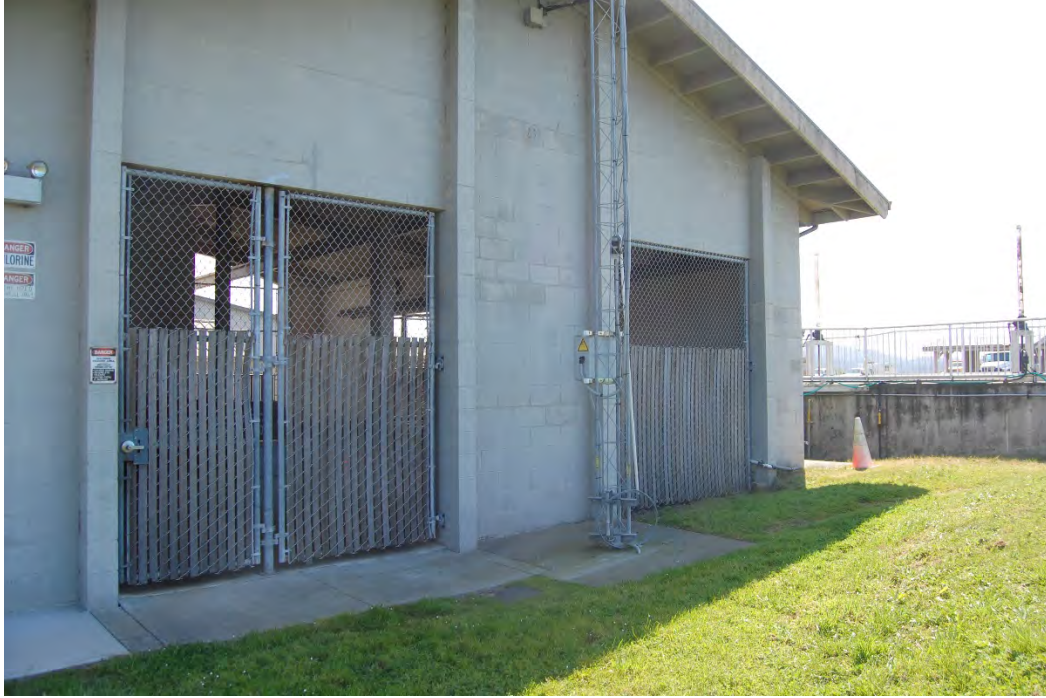
Photo 52 - Chlorine Storage Building
