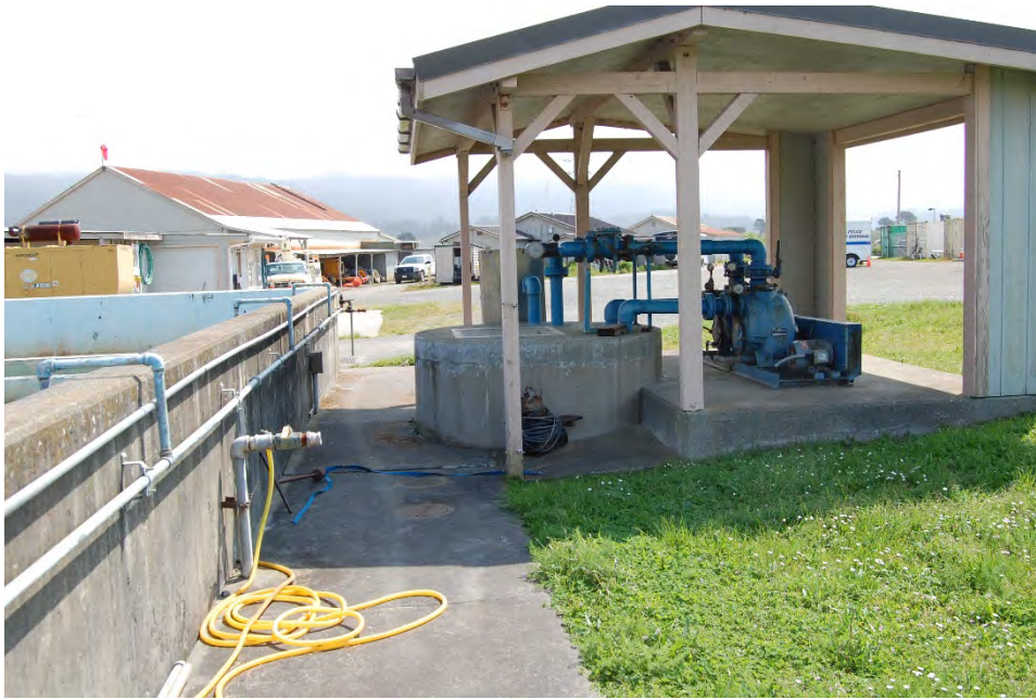
Photo 56 - Chlorine Contact Basin Drain Pump Station
