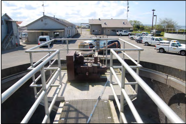
Photo 16 - Primary Clarifier No. 1 - Drive Mechanism
