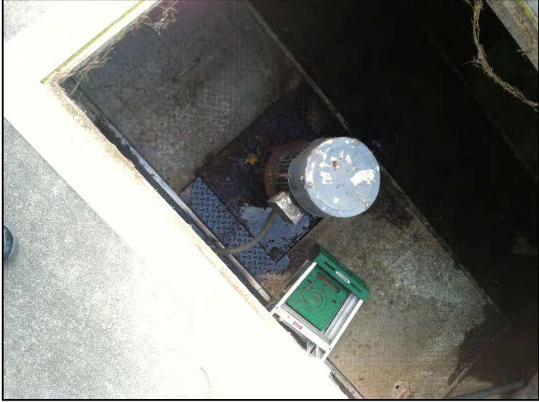
Photo 44- Enhancement Wetlands Pump Station
