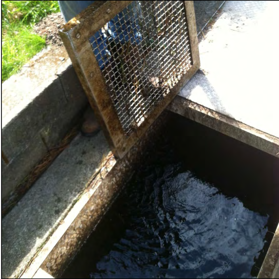
Photo 43- Enhancement Wetlands Pump Station - Inlet Manual Screen
