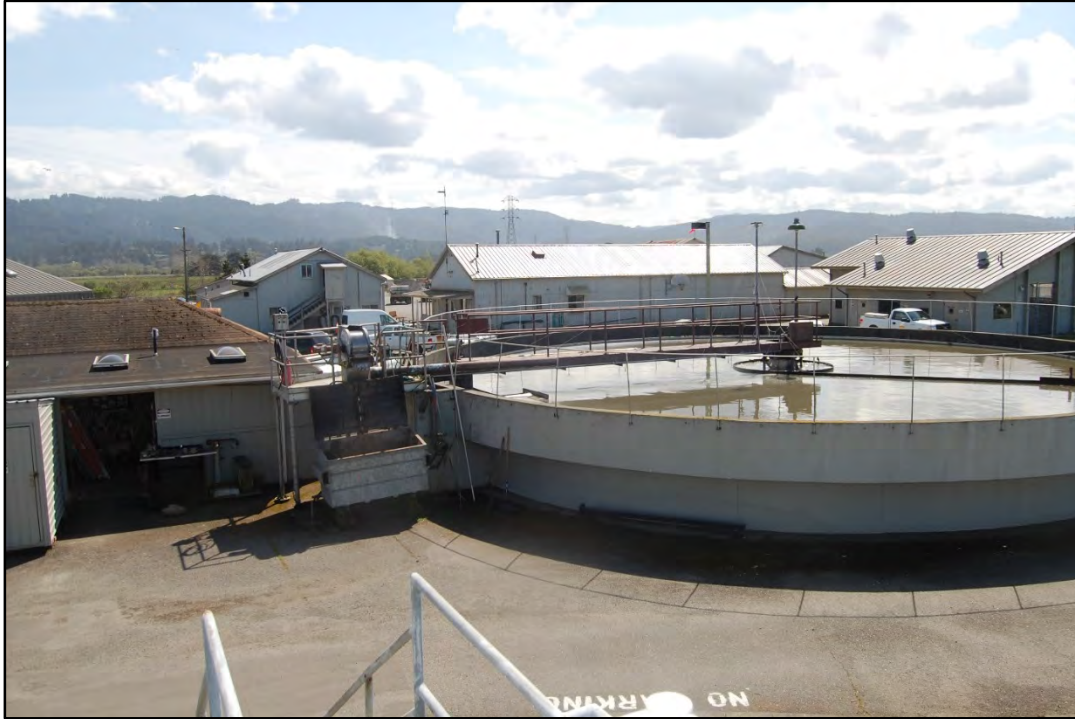
Photo 11 - Primary Clarifier No. 2 (larger unit)
