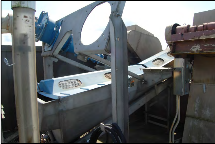
Photo 08 - Headworks Grit Classifier
