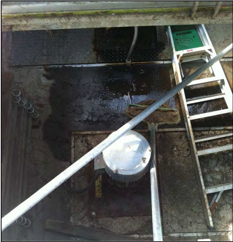
Photo 45- Enhancement Wetlands Pump Station
