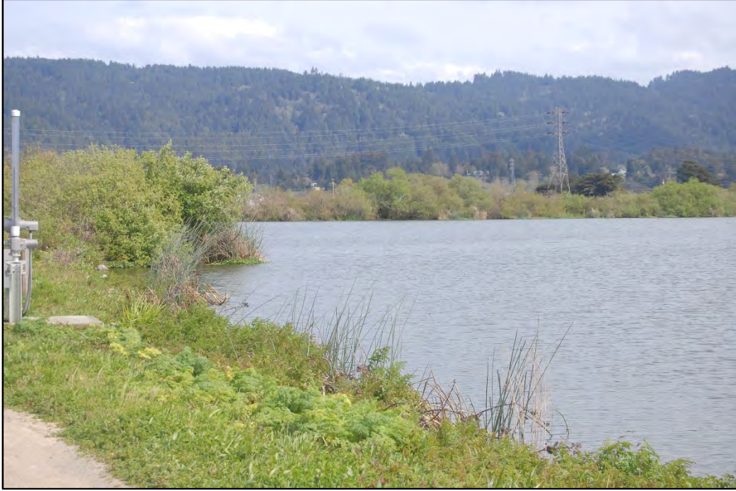
Photo 25 - Pond 2 - Outlet side and weir structure
