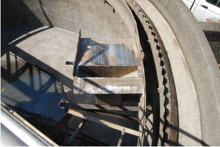
Photo 17 - Primary Clarifier No. 1 - Scum Beach and Effluent Weir
