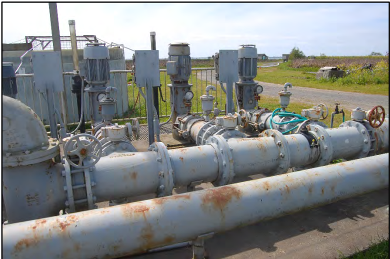
Photo 35 - Pond Pump Station and Pump Station 1
