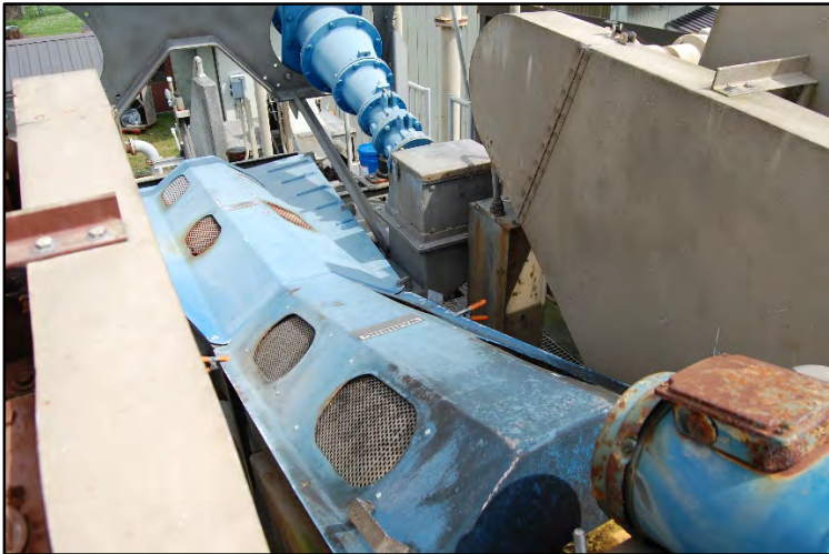
Photo 09 - Headworks Grit Classifier
