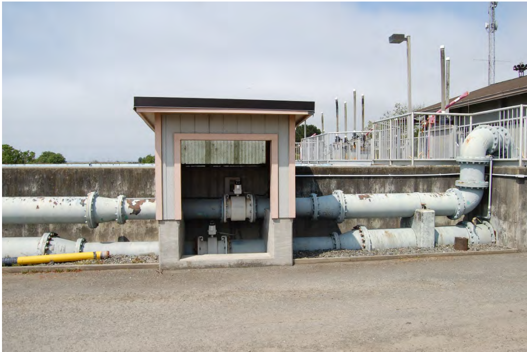
Photo 55 - Chlorine Contact Basin - Treatment wetland Influent piping and flowmeters
