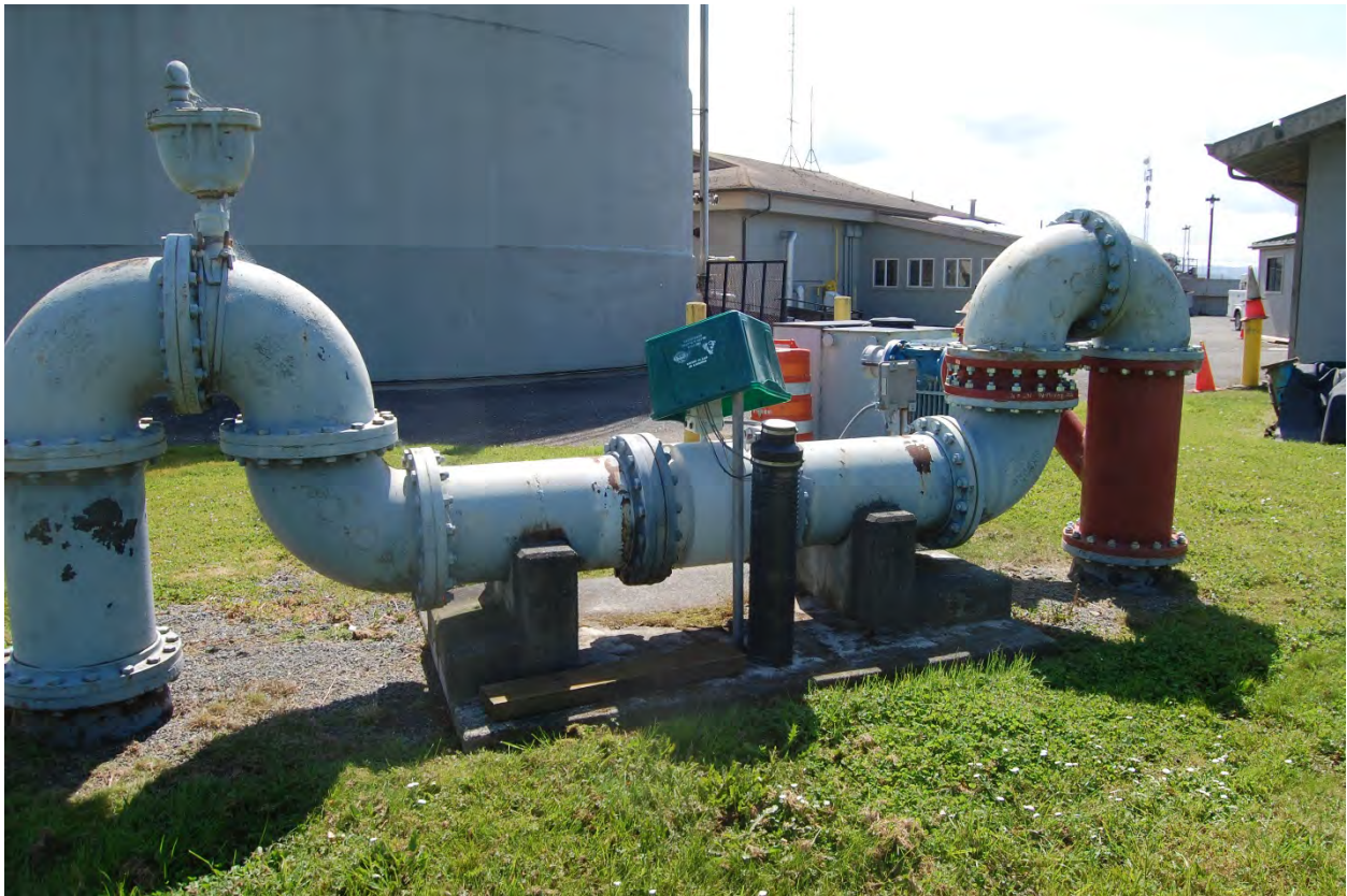
Photo 57: Bypass Flowmeter
