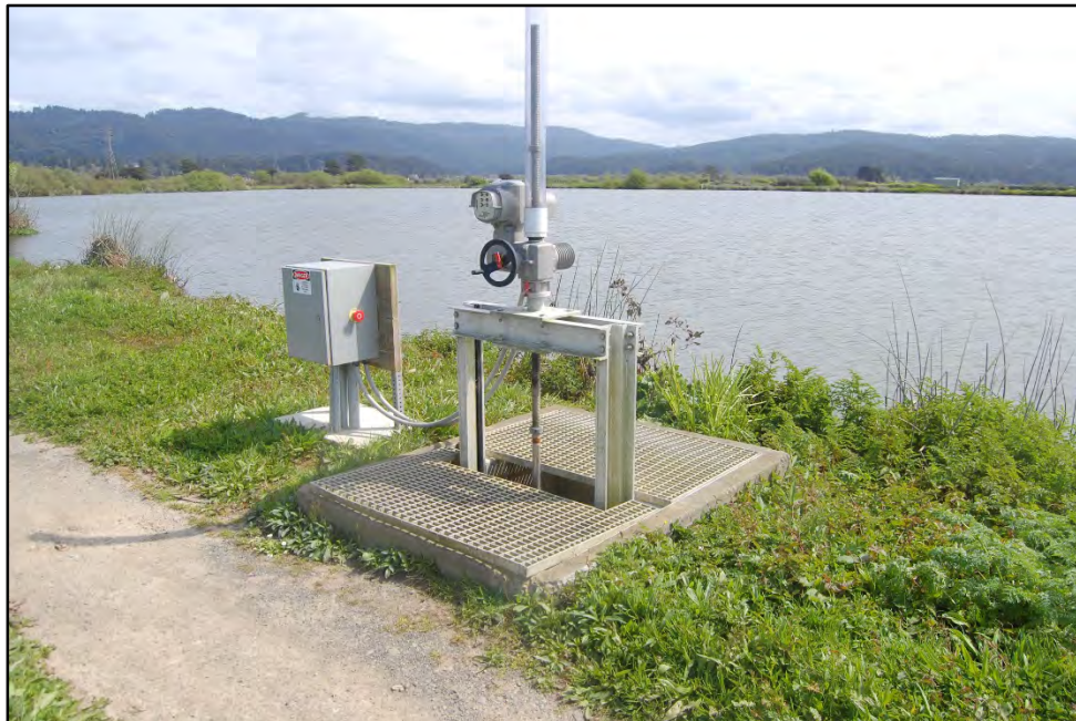
Photo 32 - Treatment Wetlands Influent Box - Automated weir
