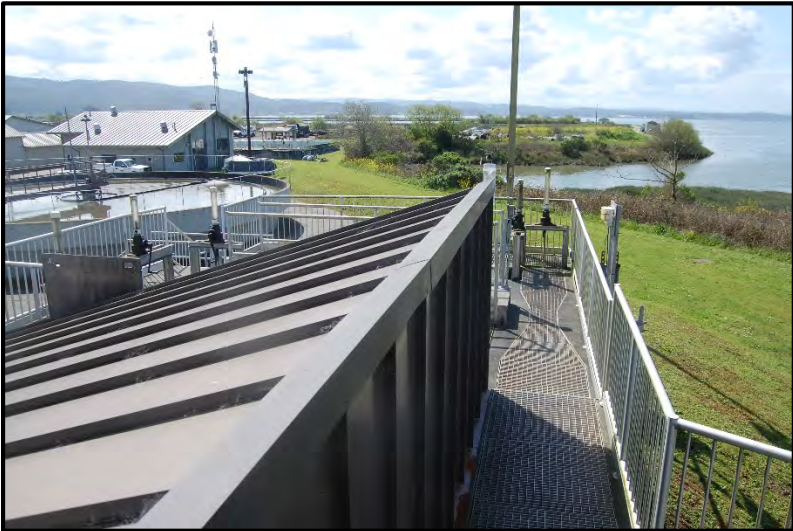
Photo 10 - Headworks - Flume Channel
