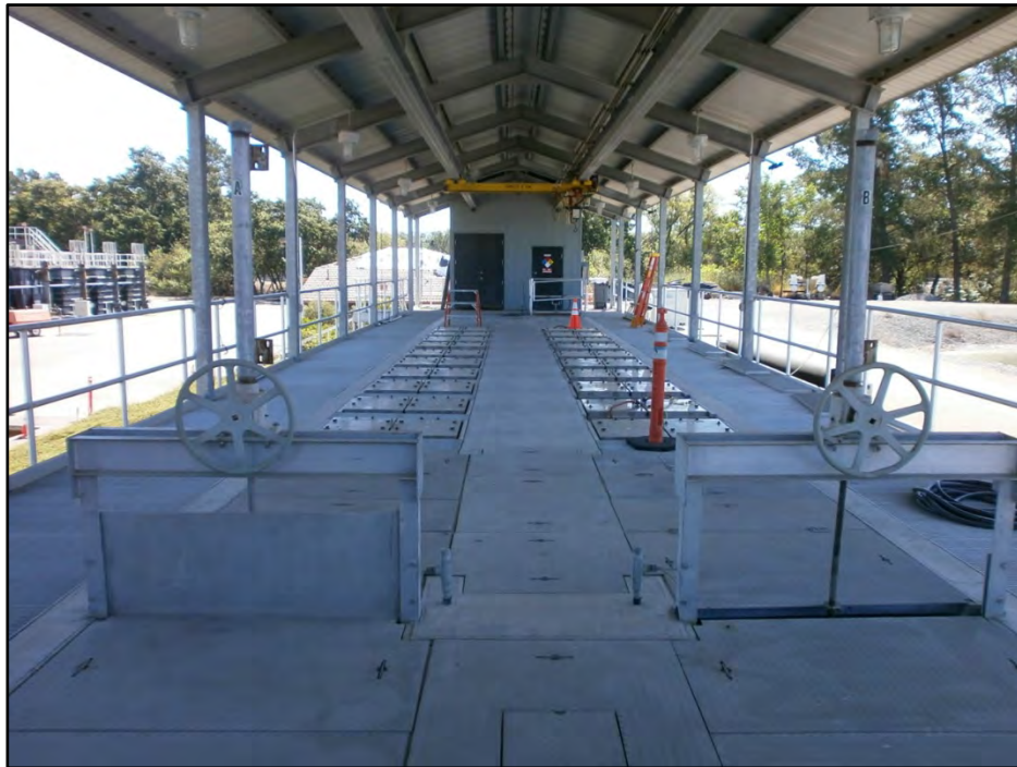
Figure 7.6 Typical Canopy Roof Over UV Channels (Windsor, California)
