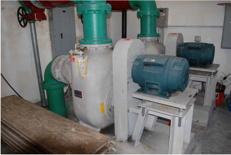
Photo 39 - Emergency Pond Pumps
