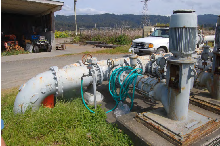
Photo 36 - Pond Pump Station and Pump Station 1
