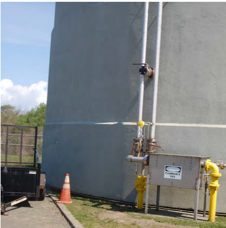
Photo 59 - Primary Digester Gas Piping
