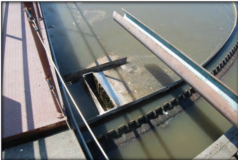
Photo 12 - Primary Clarifier No. 2 - Effluent Weir and Scum Box
