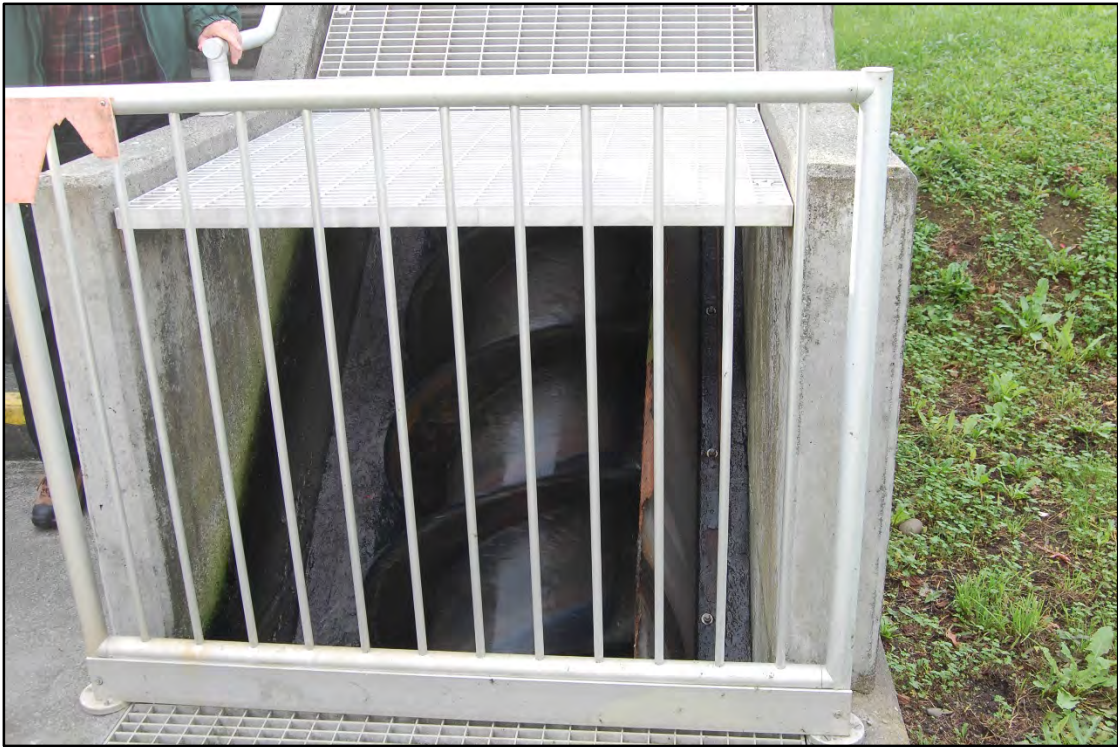
Photo 04 - Headworks - Screw Pump Close up.
