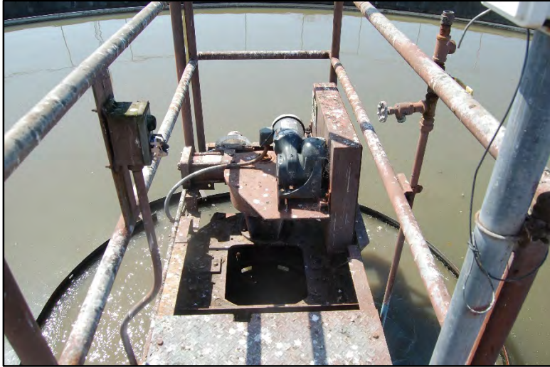
Photo 13 - Primary Clarifier No. 2 Drive Mechanism and Motor
