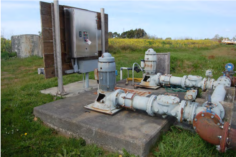
Photo 40 - Treatment Wetlands Pump Station 2 - Treatment wetlands 5 and 6
