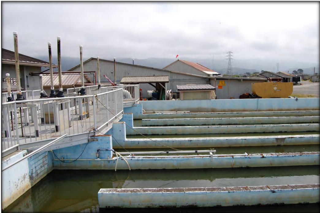
Photo 47 - Chlorine Contact Basin 2
