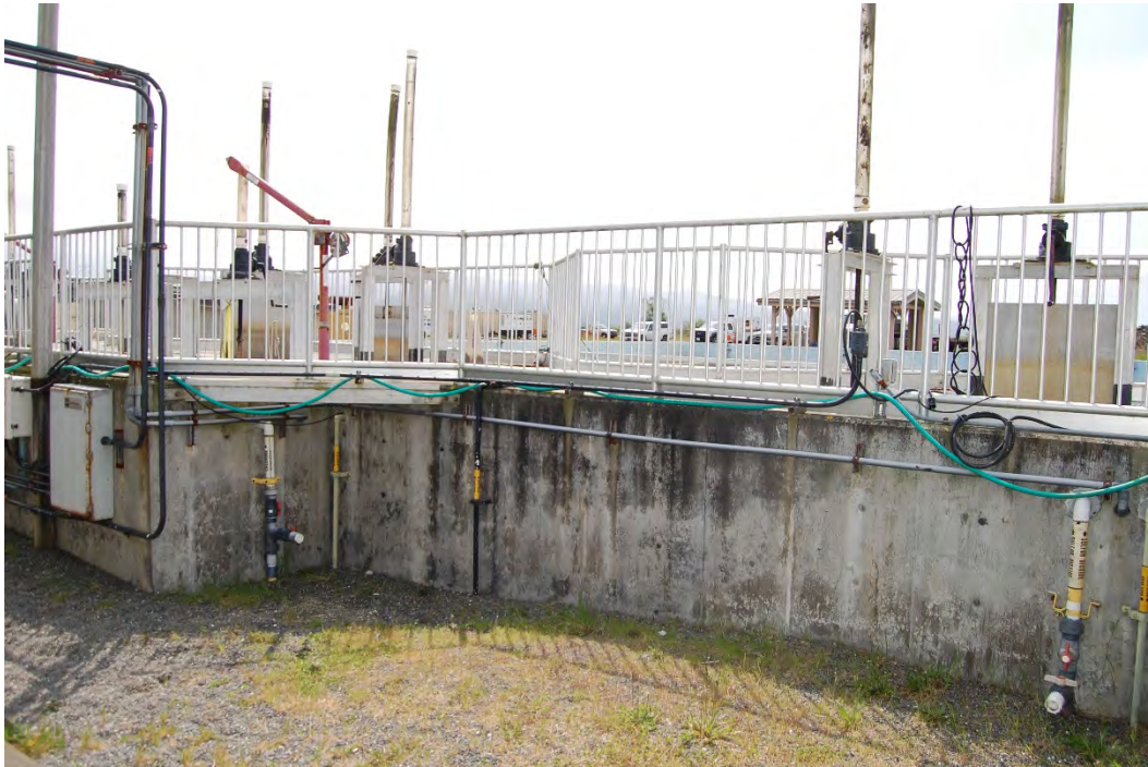
Photo 49 - Chlorine Contact Basin 3
