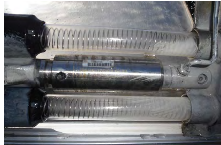
Figure 3: Visual inspection demonstrating build-up of greyish coating on area of bulbs where the wiper does not reach.
