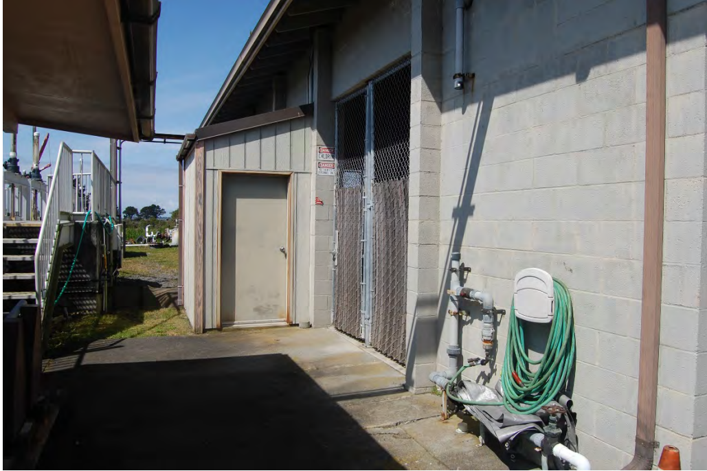
Photo 50 - Chlorine Storage Building
