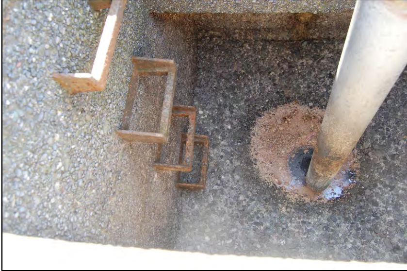
Photo 19 - Primary Clarifier No. 1 - Exposed aggregate concrete
