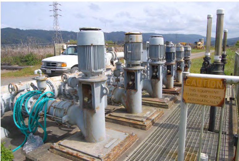
Photo 37 - Pond Pump Station and Pump Station 1
