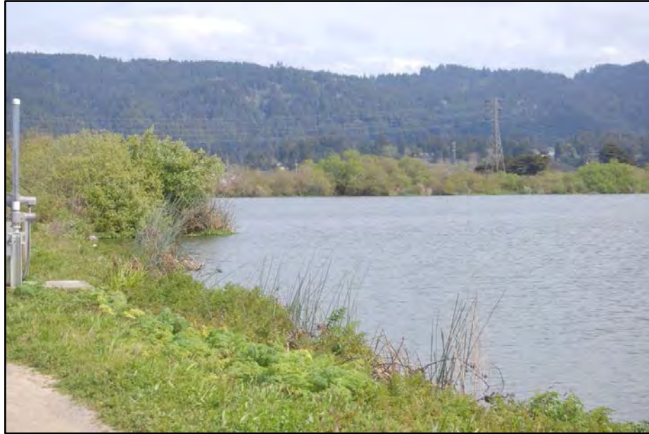
Figure 1.2 AWTF Ponds Provide Secondary Treatment
