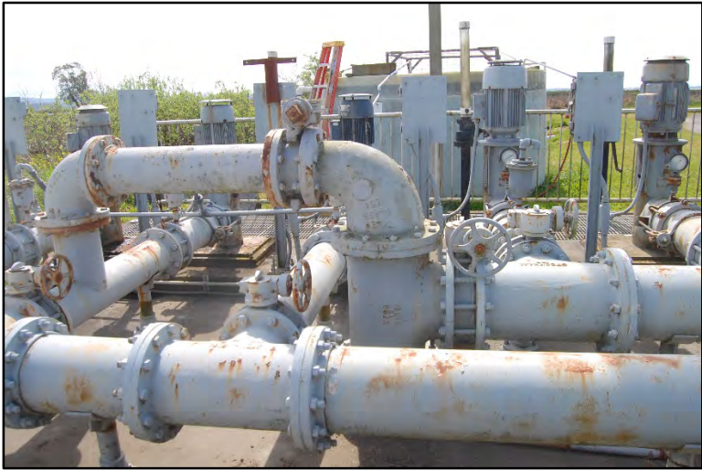
Photo 34: Pond Pump Station and Pump Station 1
