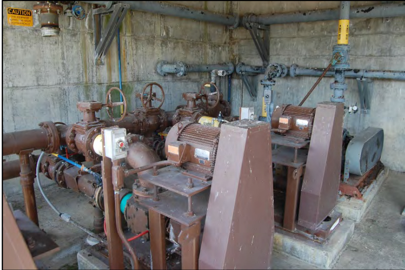
Photo 21 - Primary Clarifier Sludge Pumps
