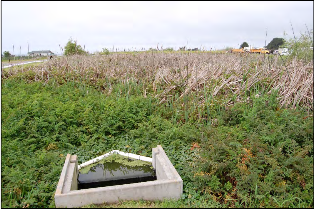
Photo 26 - Treatment wetland No. 1 - outlet structure.
