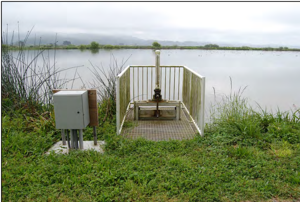
Photo 28 - Treatment Wetland 2- Inlet structure
