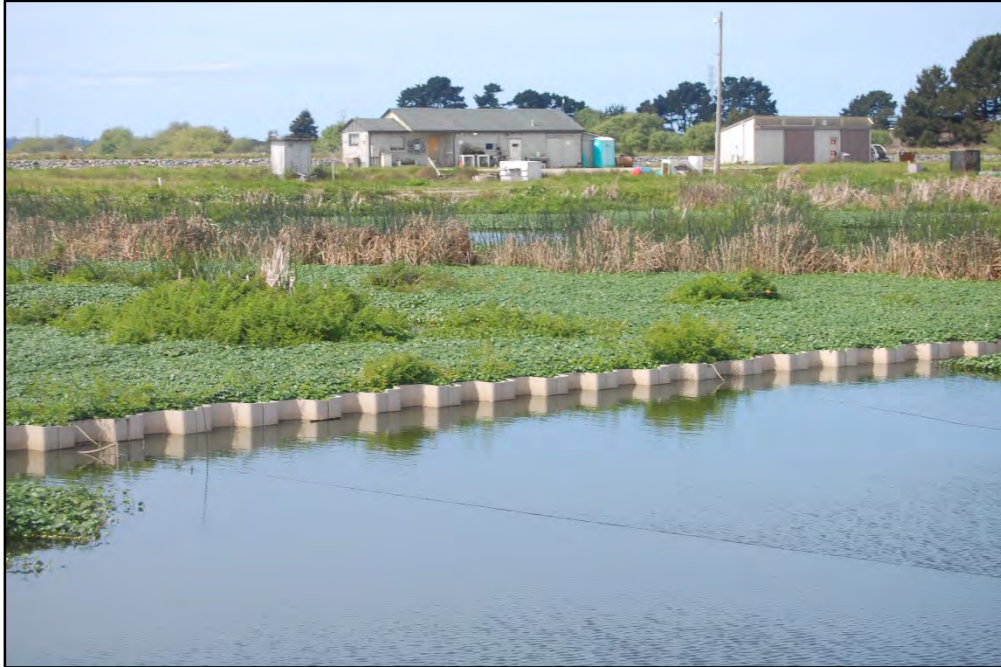
Photo 41- Treatment Wetland 4 and 5 - FRP Interlocking sheets
