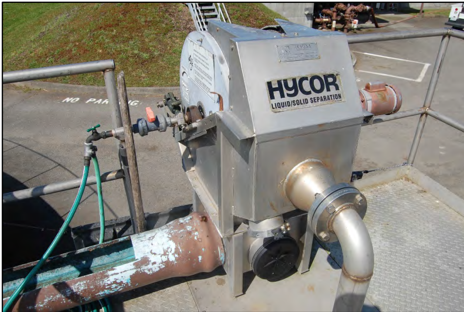
Photo 14 - Primary Clarifier No. 2 - Hycor Grease and Scum Concentrator Unit
