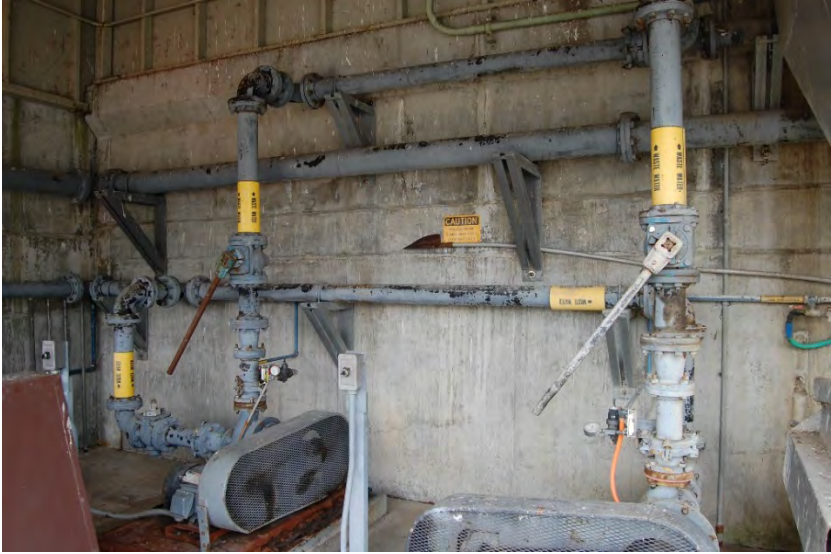
Photo 05 - Headworks Grit Pump Room
