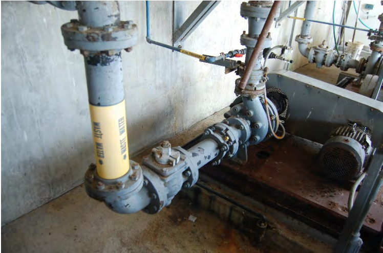
Photo 06 - Headworks Grit Pump
