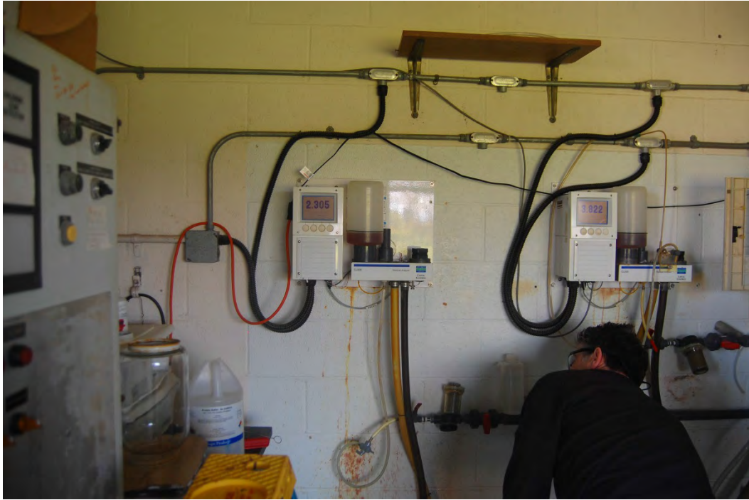
Photo 54 - Chlorine residual analyzers
