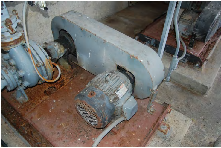
Photo 07 - Headworks Grit Pump
