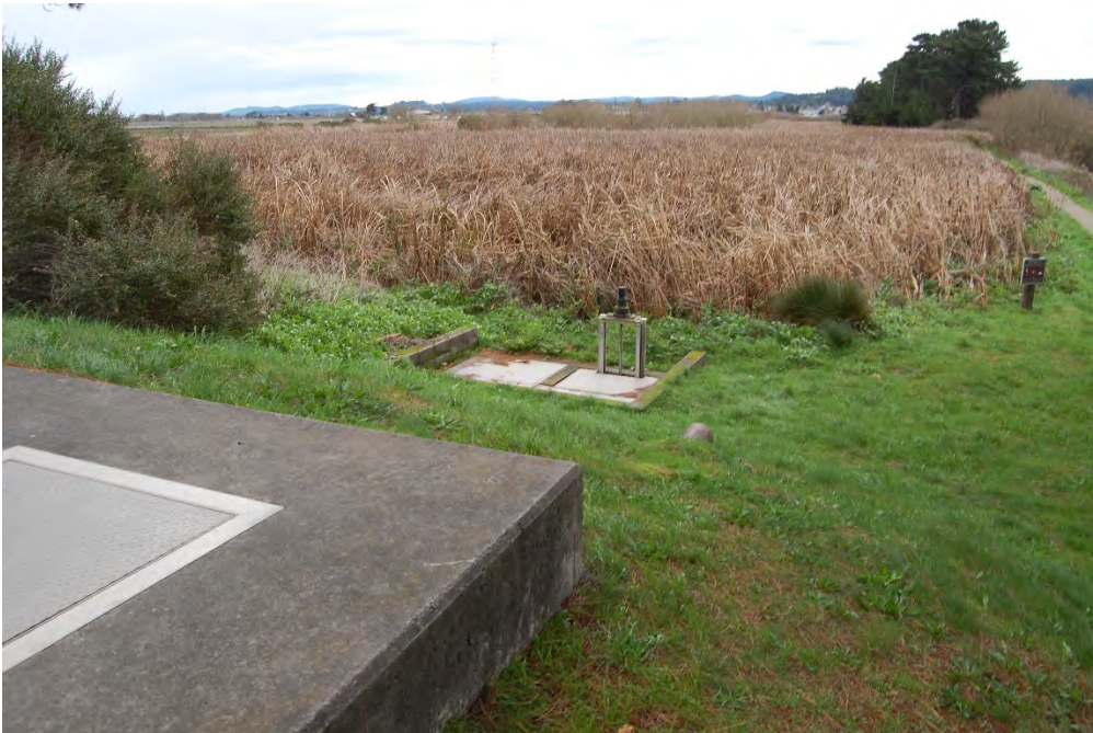
Photo 42 - Hauser Wetland Pump Station - Inlet Structure
