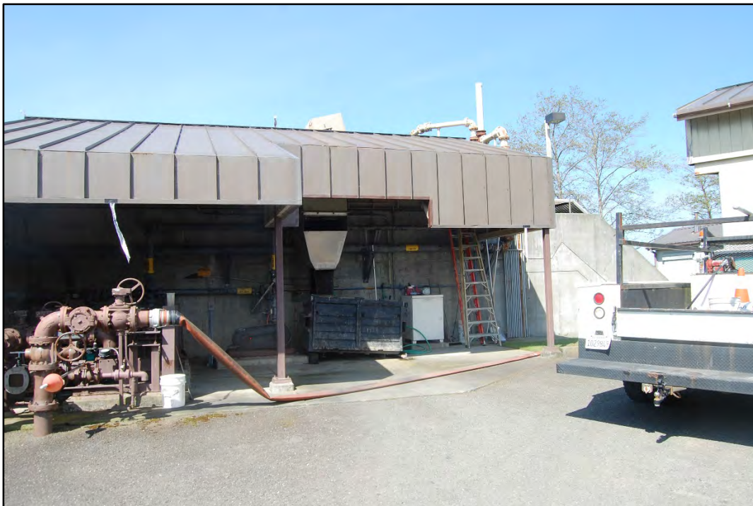
Photo 2 - Headworks - Grit Pumps, Screenings, and Grit Bin
