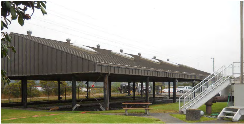
Photo 60 - Sludge Drying Beds
