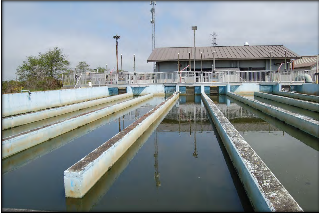
Photo 46 - Chlorine Contact Basin 1
