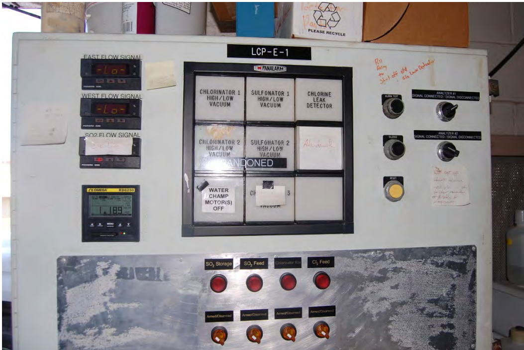
Photo 53 - Chlorine Contact Basin LCP
