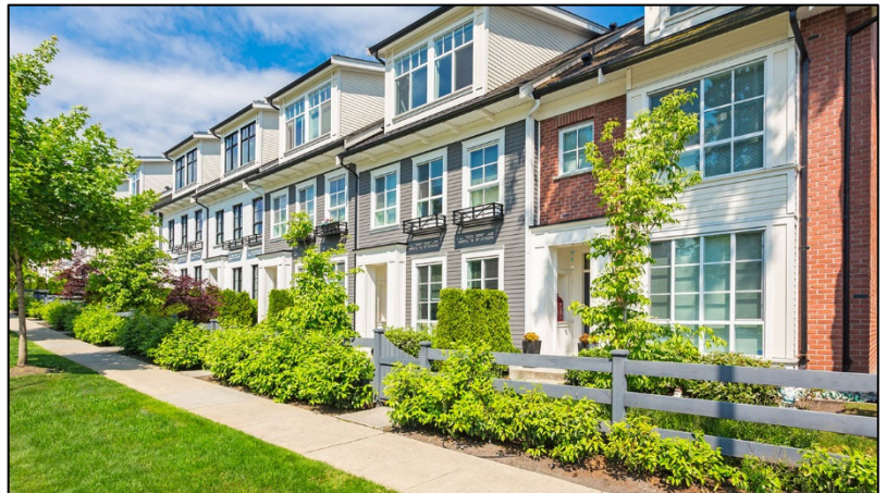
Entrances to individual units facing the street
