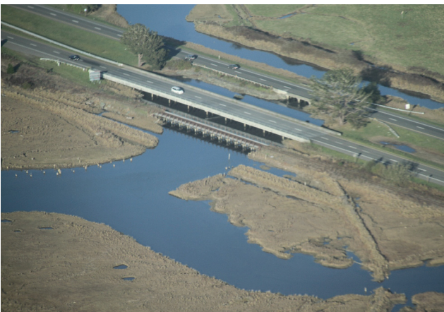
Aerial view looking northeast of Gannon Slough Bridge and Highway 101
