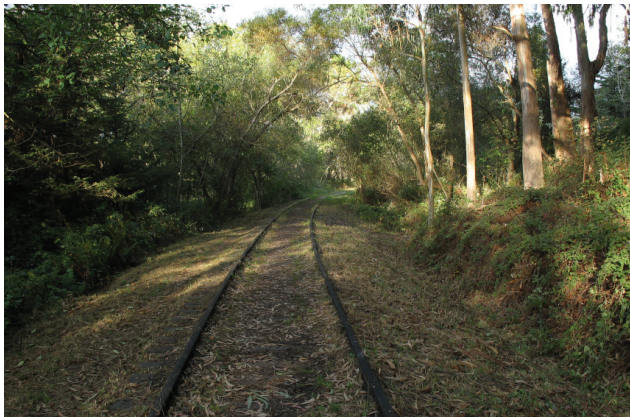
View of rail corridor looking east
