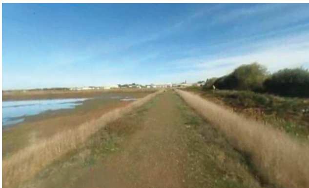
Looking north from atop the levee with existing dirt trail
