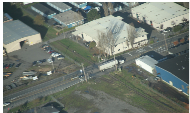
Aerial View of Samoa Blvd looking northeast
