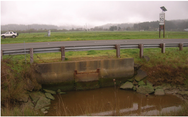
Jacoby Creek drainage culvert
