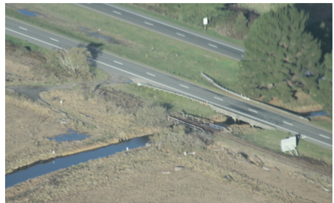
Aerial view of Jacoby Creek Bridge
