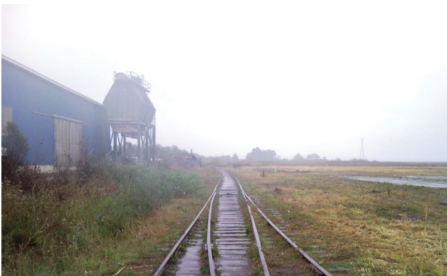
Looking south just past Samoa Blvd with industrial buildings to the east of tracks
