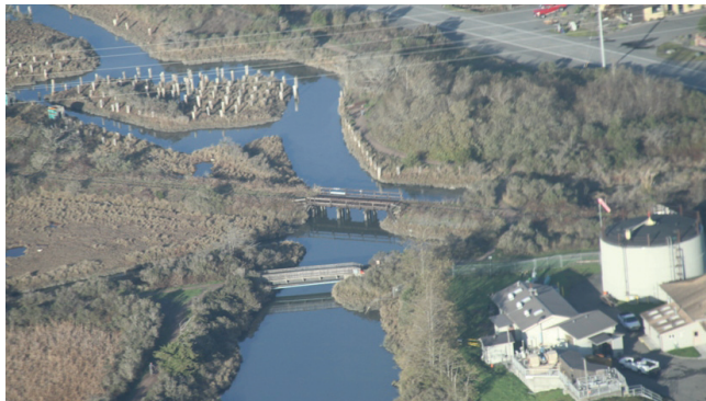
Aerial view to the northeast of pedestrian bridge and railroad bridge (background) at Jolly Giant Creek
