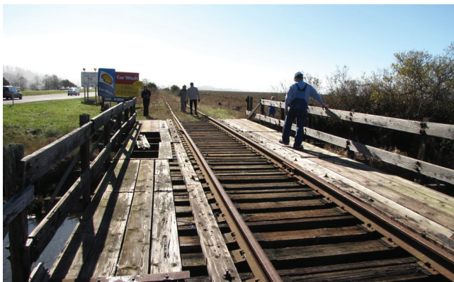
Closup view of Jacoby Creek Bridge looking south
