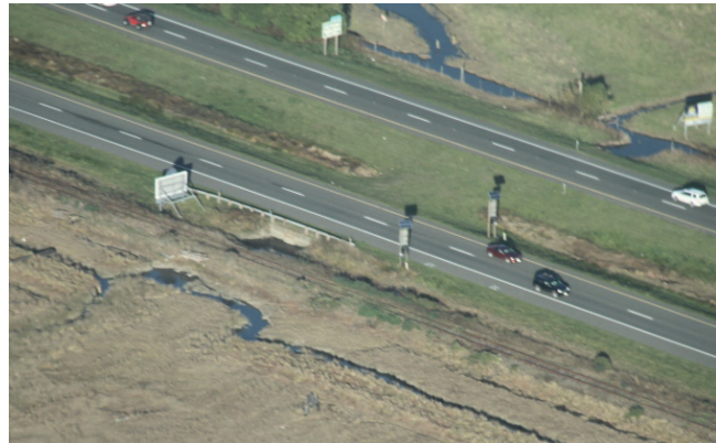
Aerial view of drainage culvert looking northeast
