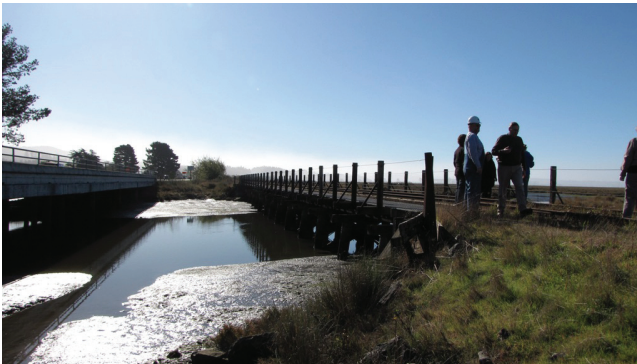
Gannon Slough railroad bridge with context of highway bridge on left
