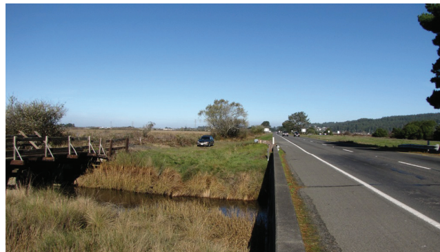
Jacoby Creek Bridge looking northwest with Highway 101 context
