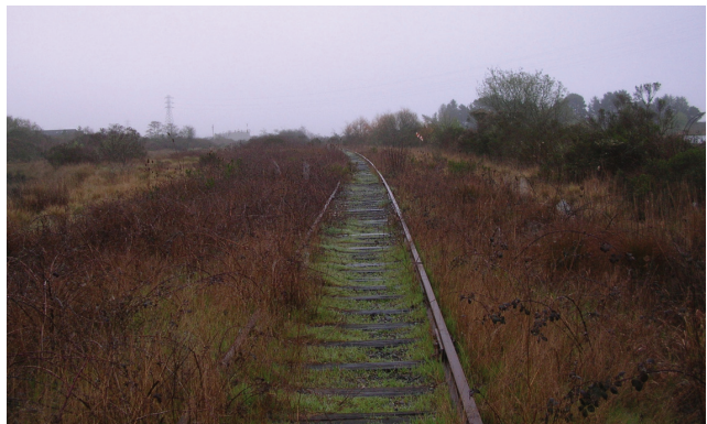
View of rail corridor south of I Street looking south
