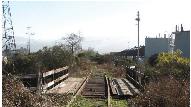
Looking southeast on railroad bridge at Jolly Giant Creek
