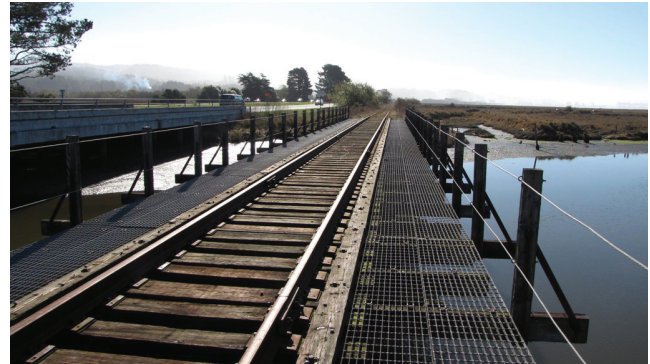
Gannon Slough Bridge looking south
