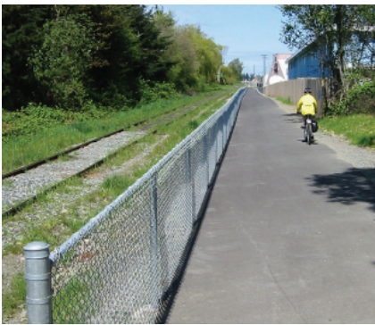
Fencing separates a multi-use trail from an active rail corridor.
