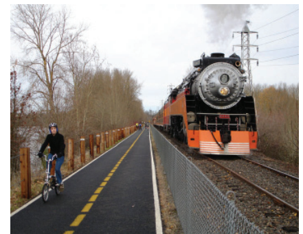
A popular RWT showing 8.5' minimum setback from edge of trail to rail centerline
