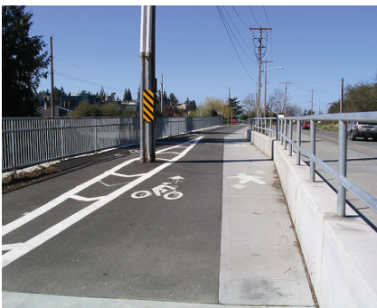
Pathway obstructions should be avoided. However, they should be clearly marked in areas where they must occur
