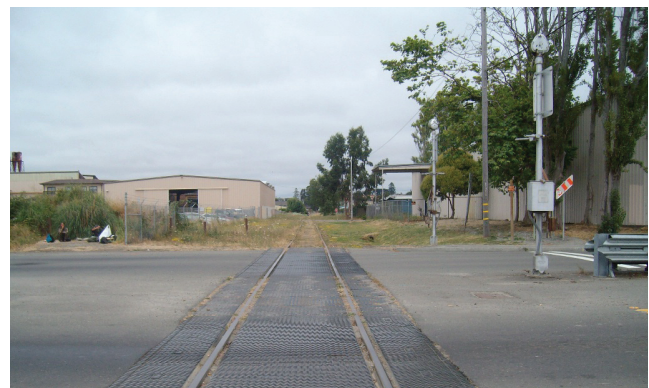
Tracks across Samoa Blvd looking north
