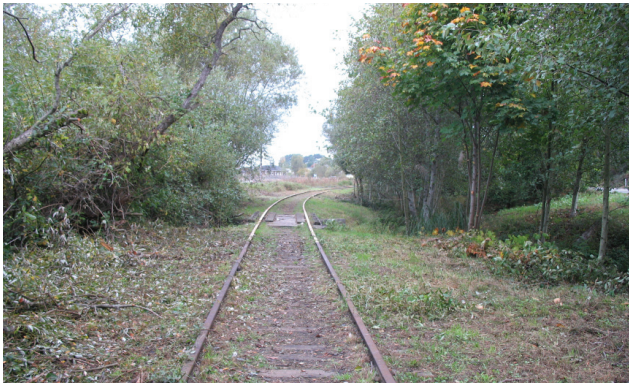
View of rail corridor looking north
