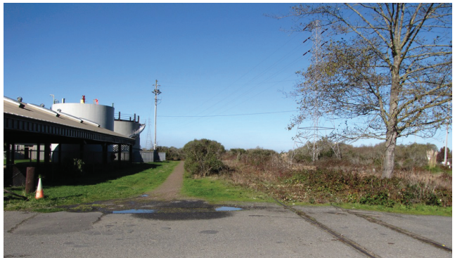
Existing dirt trail and railroad looking northwest from Waste Water Treatment Plant Driveway
