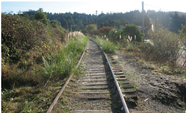
View of rail corridor near Sunset Avenue looking east
