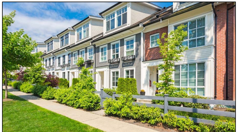
Entrances to individual units facing the street
