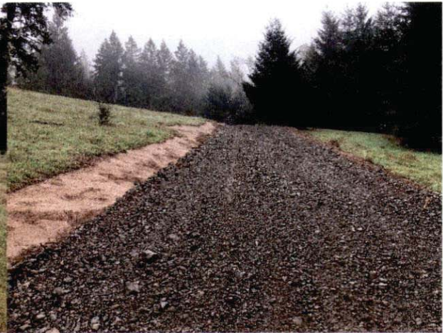
Photo #10 Access Road Looking Southwest
