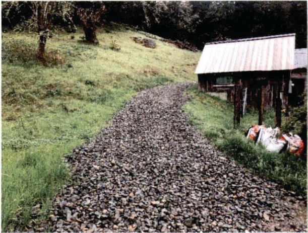
Photo #29 Access Road Looking South
