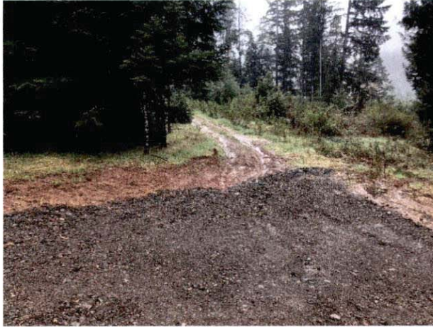
Photo #13 Access Road Looking South
