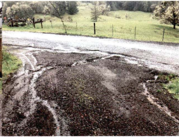
Photo #34 @ Alderpoint Rd & Driveway Looking West
