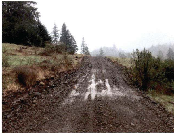
Photo #16 Access Road @ Cultivation Looking South
