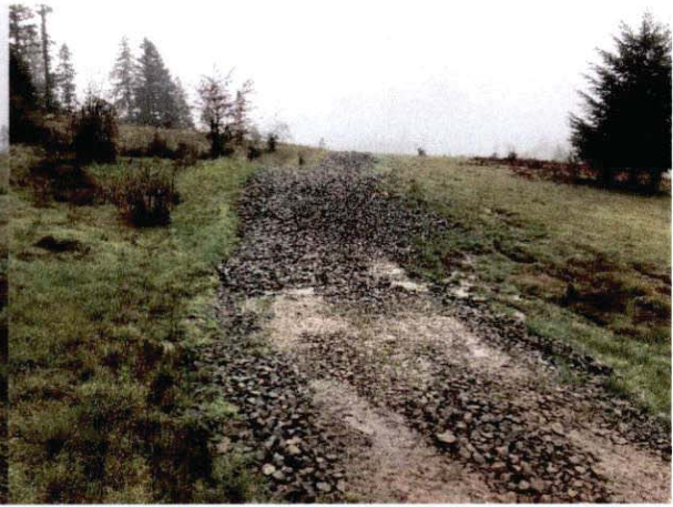
Photo #8 Access Road Looking South
