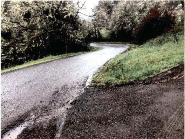
Photo #35 Alderpoint Rd & Driveway Looking North
