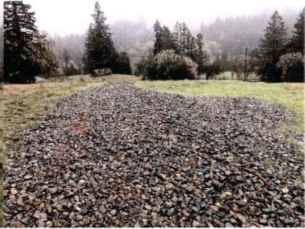
Photo #20 Access Road Looking South
