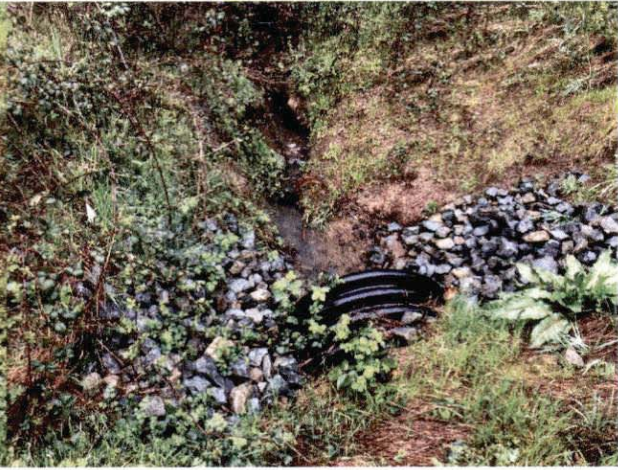
Photo #28 Culvert Inlet
