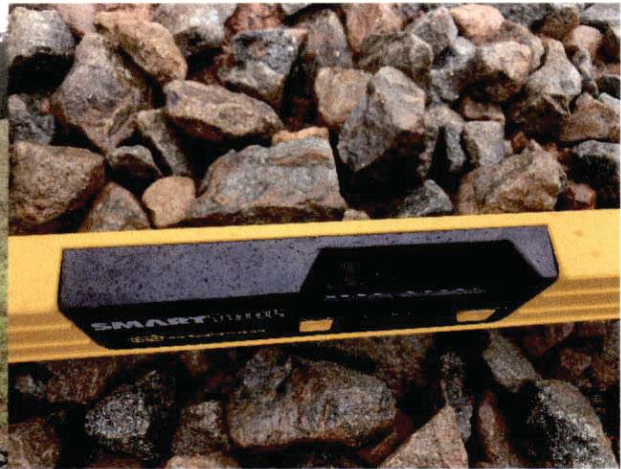
Photo #22 Grade on Access Road
