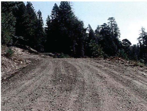
Figure 38. Pinchard Creek road immediately after project construction, 2002. Photo: Joe Hoffman, Plumas National Forest.
