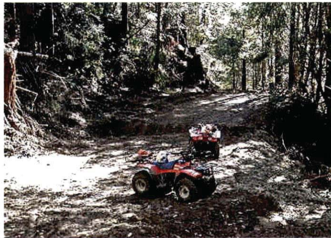
Figure 9. Water bars installed on a road after timber harvesting. Source: Angela Wilson, Central Valley Regional Water Quality Control Board.
