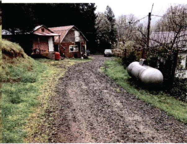
Photo #32 Access Road Looking Southwest
