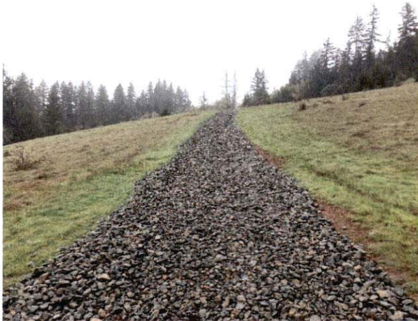
Photo #21 Access Road Looking North Towards Cultivation
