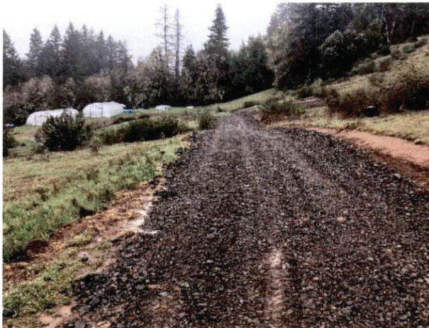
Photo #17 Access Road Looking North Towards Cultivation
