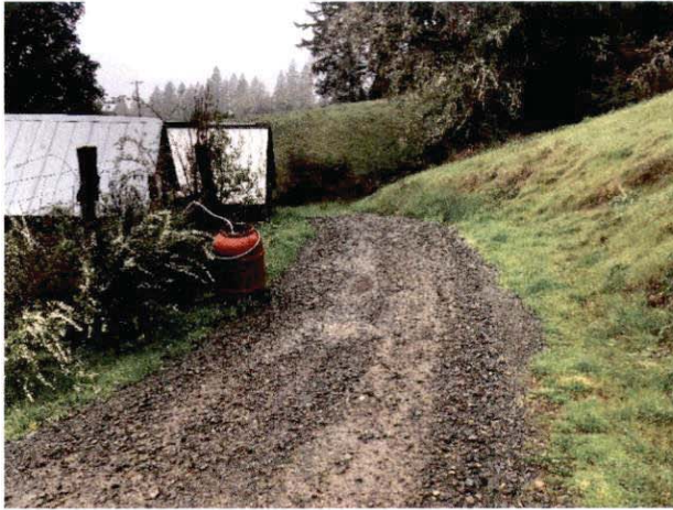
Photo #31 Access Road Looking North
