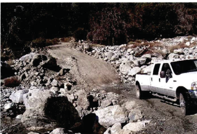
Figure 6. Low-water crossing on a perennial stream, San Bernardino County. Photo: Richard Harris.
