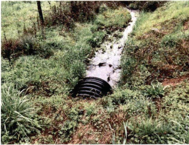
Photo #27 Culvert Discharge
