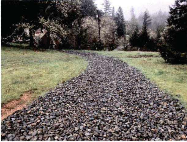
Photo #25 Access Road Looking South
