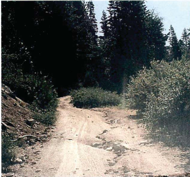
Figure 37. Pinchard Creek road with rilling along the road surface before the project, 2002. Photo: Joe Hoffman, Plumas National Forest.
