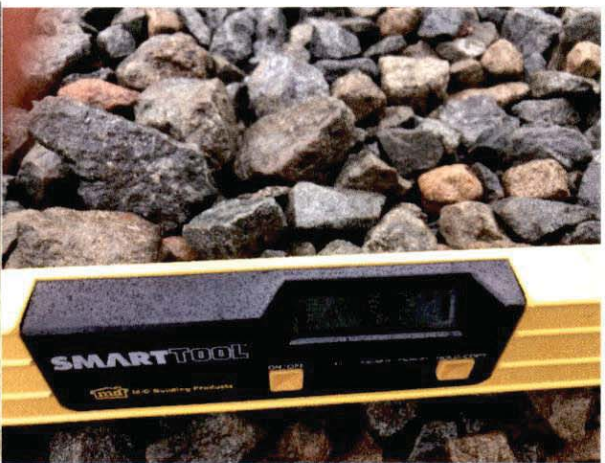
Photo #24 Grade on Access Road
