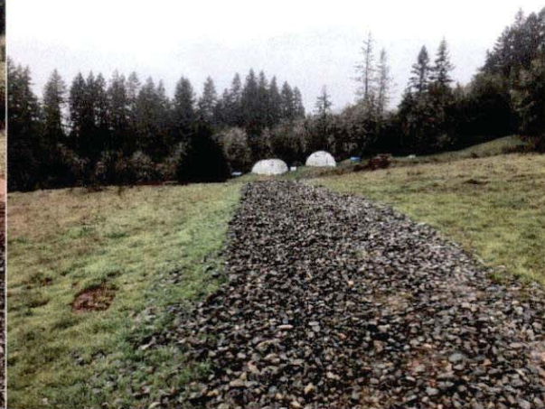
Photo #18 Access Road Looking North Towards Cultivation
